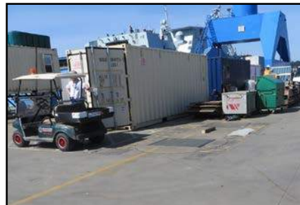
AUTHORIZED Sanitary Sewer Discharge point, Lift Station #15.
