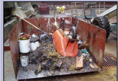
INADEQUATE waste grit storage.
