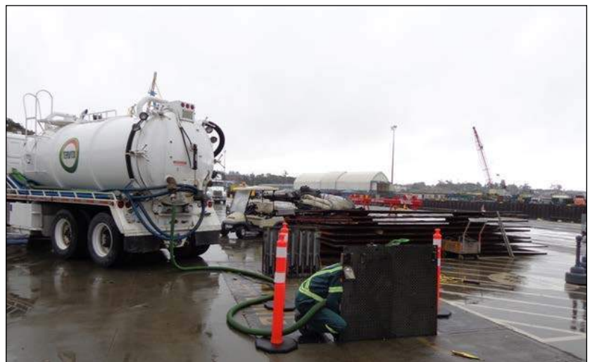
Lift Station Maintenance.
