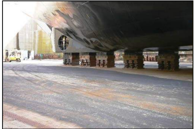
INADEQUATE: Example of a dock floor that would not pass inspection.
