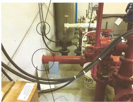
PIPE THROUGH WALL TO BE REMOVED. WALL OPENING TO BE FILLED WITH INSULATION AND INTERIOR REPAIR TO MATCH EXISTING. PROVIDE PAINTED WOOD COVERING ON OUTSIDE OPENING AND SEAL AS REQUIRED TO MAKE WATER TIGHT. (TYP. AT 2 LOCATIONS)
