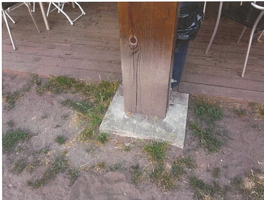
Photo #2: Shallow Foundation for Column supporting existing Canopy
