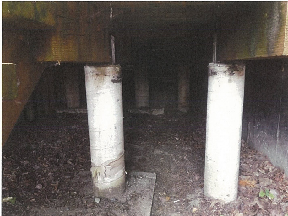
Photo #4: Sonnet Tube supporting the timber deck
