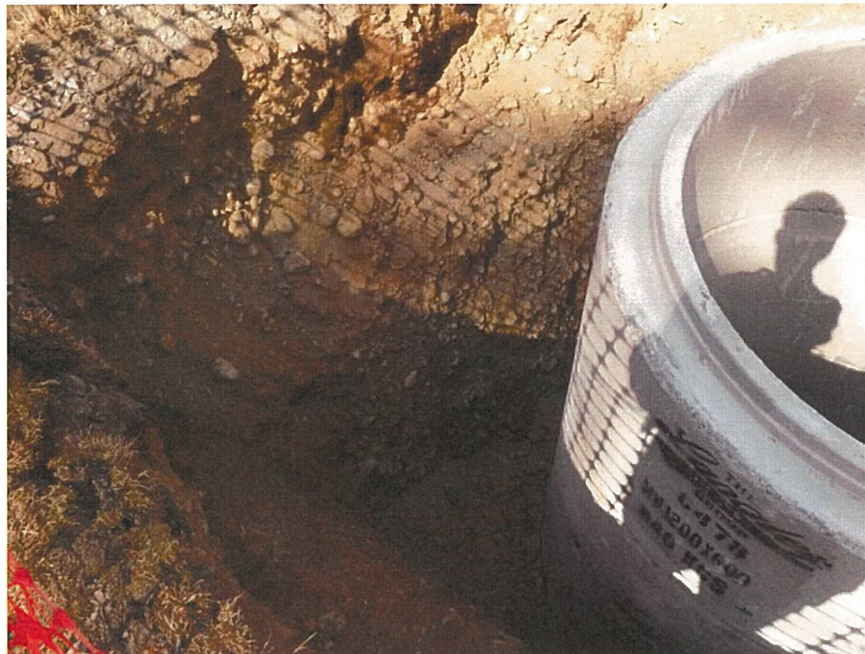
Photo #6: Nearby Drainage Construction identify dense SAND and Gravel in Excavation
