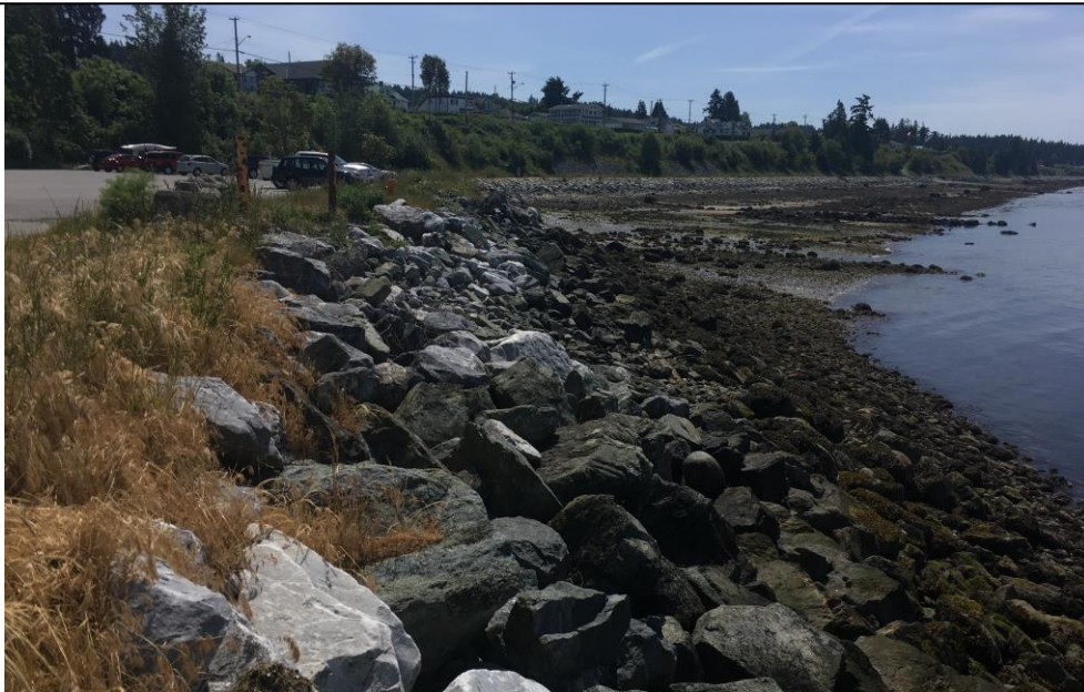
Photo 4: Typical existing rip rap foreshore erosion protection looking southwest along the south edge of the site. This is illustrative of the potential nature of some of the buried fill.
