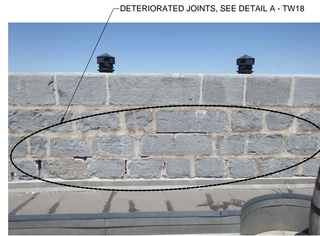
PHOTO 1 CHIPPING & REPOINTING - WEST ELEVATION
