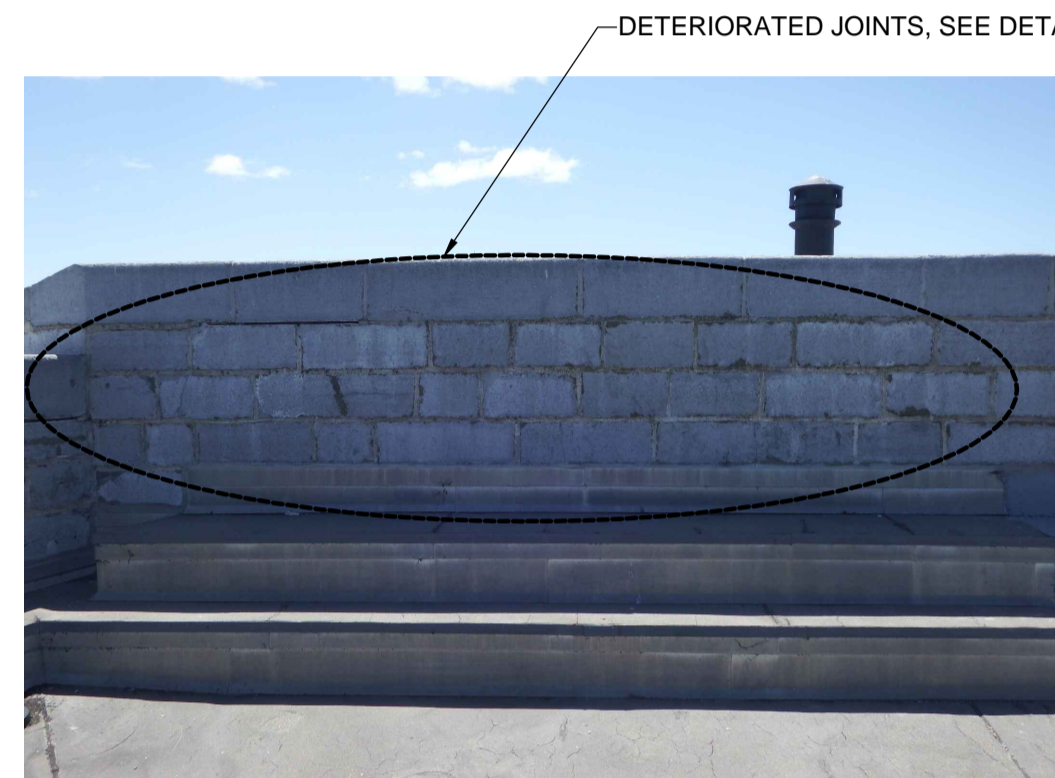
PHOTO 3 CHIPPING & REPOINTING - SOUTH WEST ELEVATION
