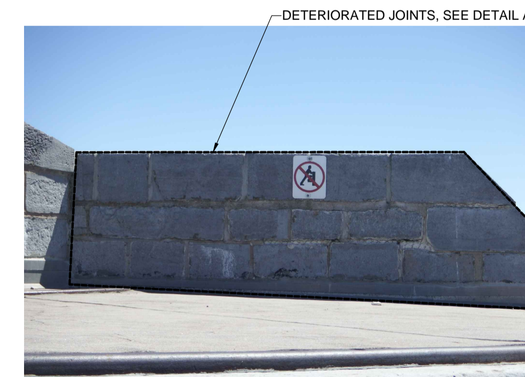
PHOTO 8 CHIPPING & REPOINTING - EAST ELEVATION
