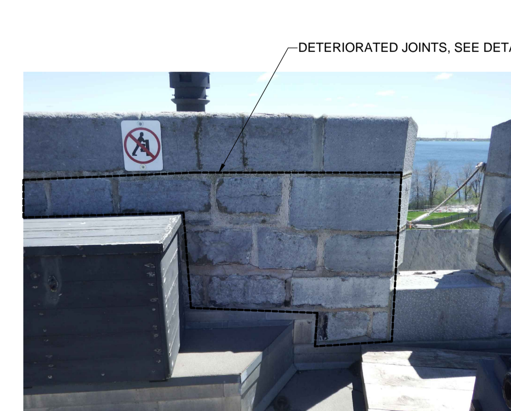
PHOTO 12 CHIPPING & REPOINTING - EAST ELEVATION
