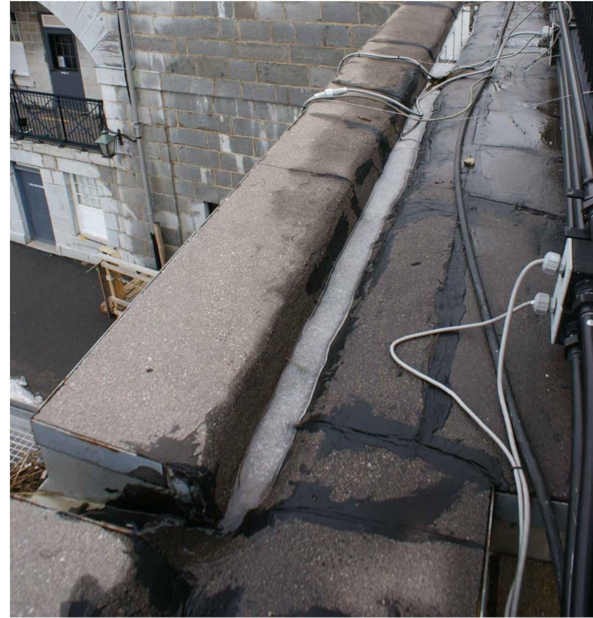
MASTIC ASPHALT GUTTER AT BLOCK 04 THROUGH 09 N.T.S.
