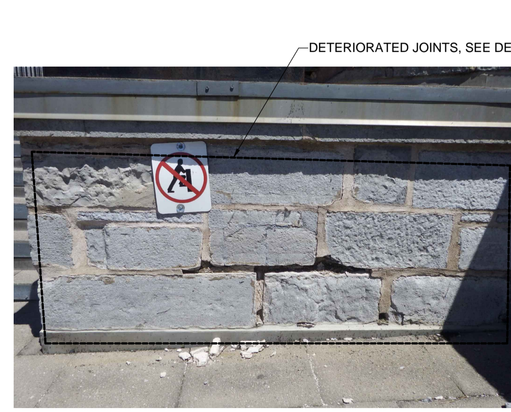
PHOTO 11 CHIPPING & REPOINTING - EAST ELEVATION
