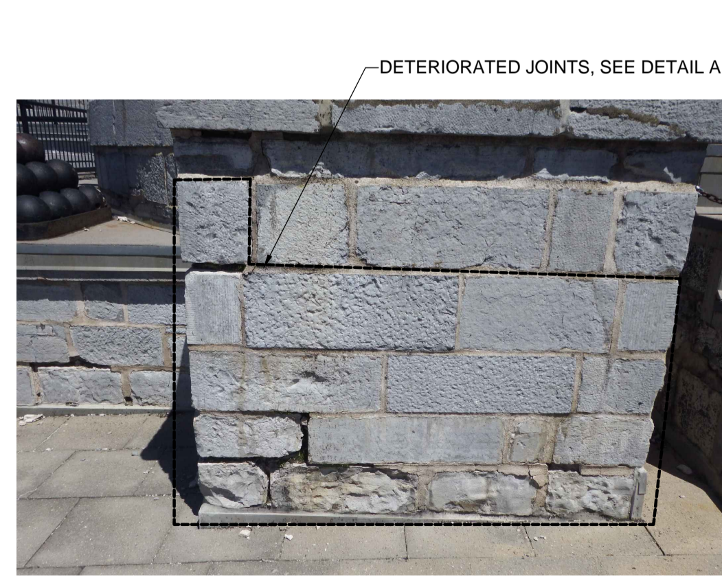
PHOTO 10 CHIPPING & REPOINTING - EAST ELEVATION
