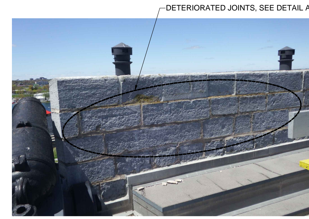
PHOTO 2 CHIPPING & REPOINTING - WEST ELEVATION
