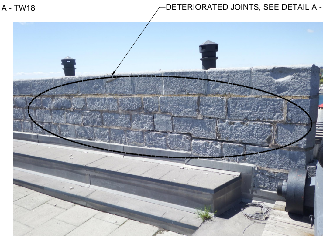
PHOTO 4 CHIPPING & REPOINTING - WEST ELEVATION
