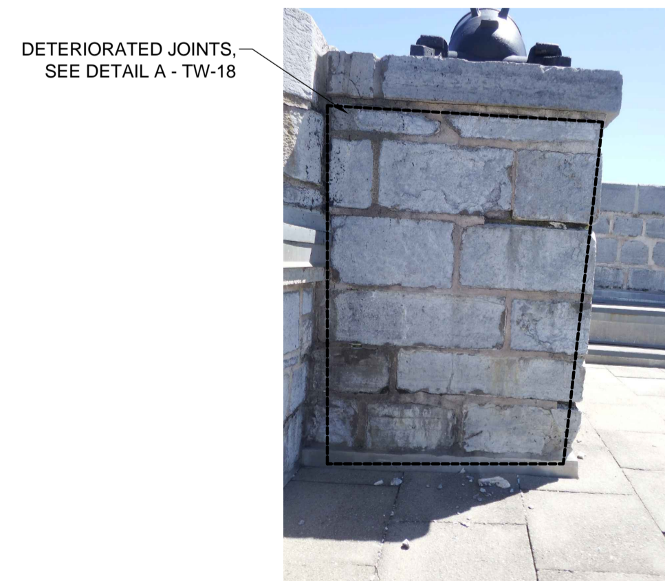
PHOTO 9 CHIPPING & REPOINTING - EAST ELEVATION
