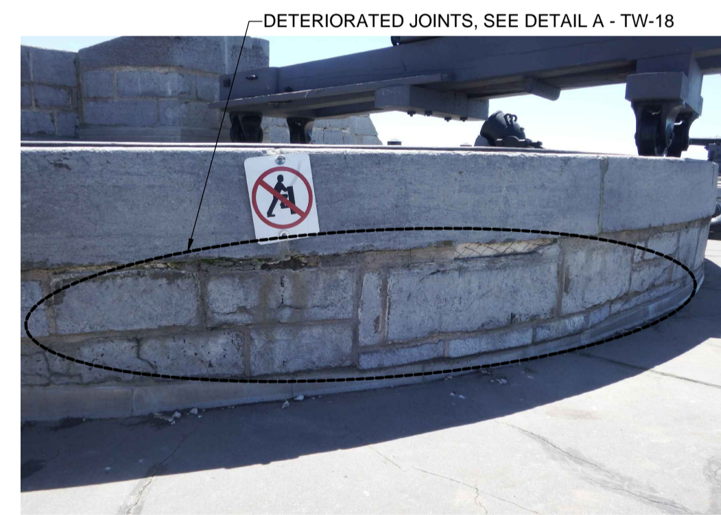
PHOTO 7 CHIPPING & REPOINTING - EAST ELEVATION
