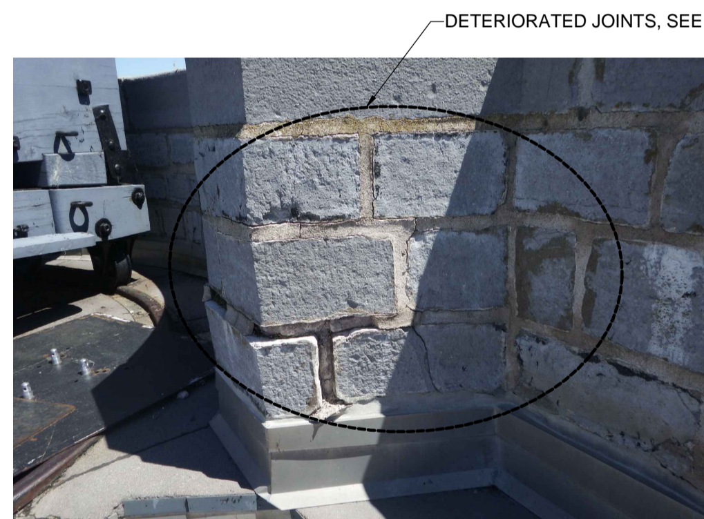
PHOTO 5 CHIPPING & REPOINTING - EAST ELEVATION
