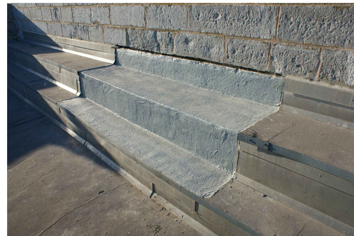
MOCK-UP AREA WITH FLASHING REMOVED N.T.S.
