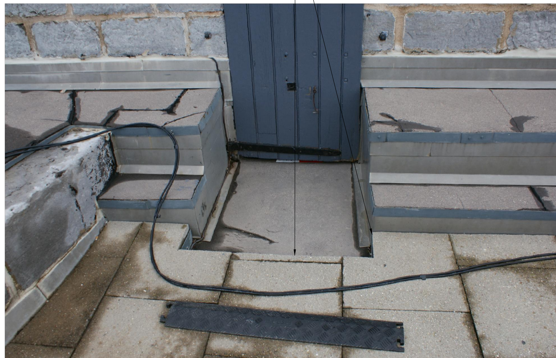
DOORWAY OPENING AT FIRING STEPS
