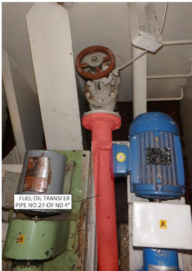
Figure 18 Fuel Oil Transfer 27-OF, connection at longitudinal bulkhead
