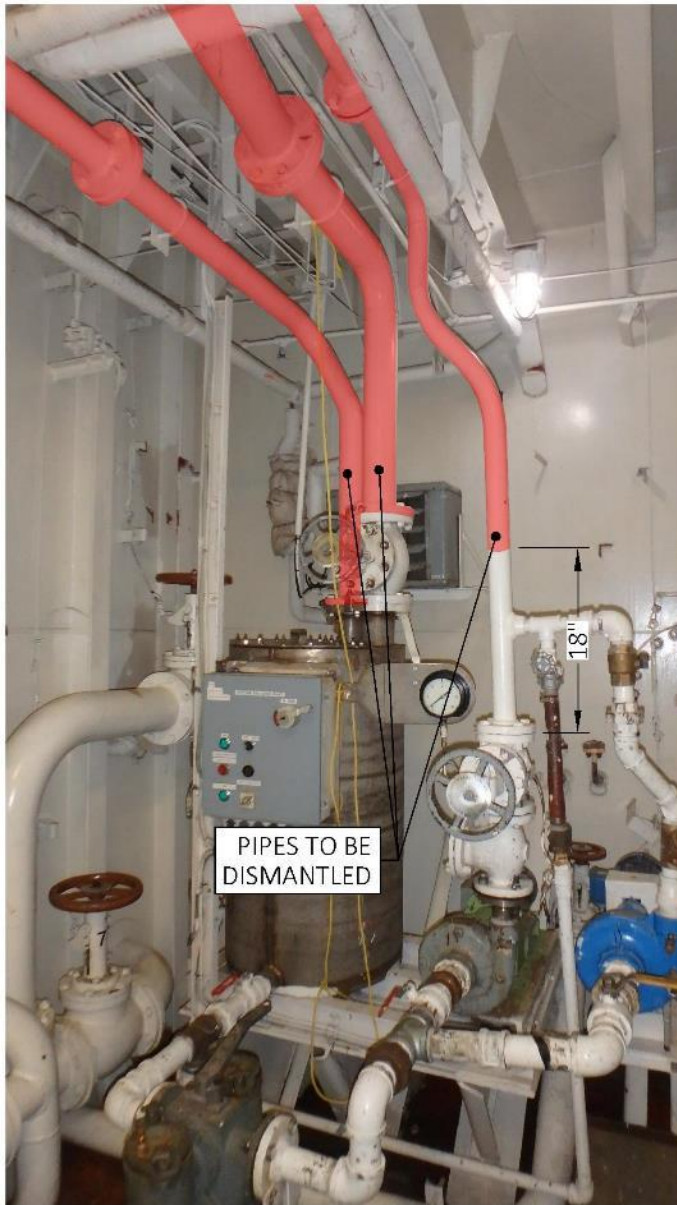
Figure 26 Grey water system
