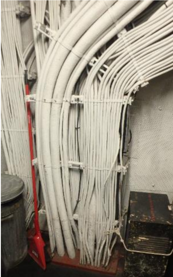
Figure 36 Vertical route in static inverter compartment
