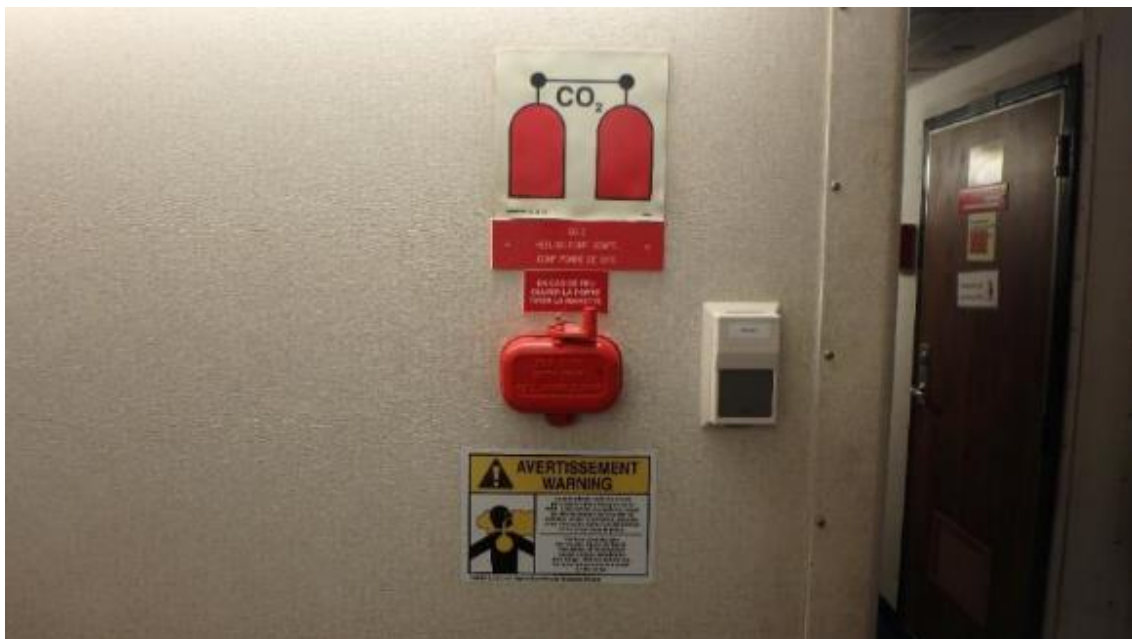
Figure 6 CO2 Pull Box Station, frame 139, main deck starboard
