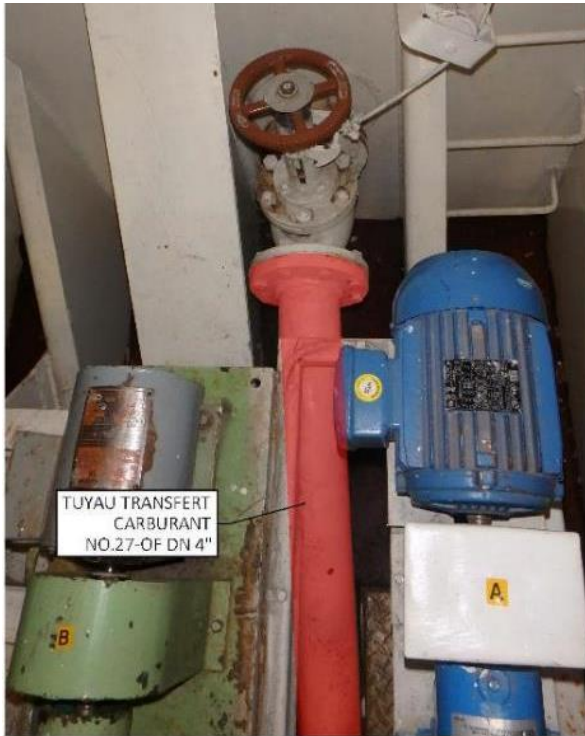
Figure 18 Transfert de carburant 27-OF, raccord à la cloison
