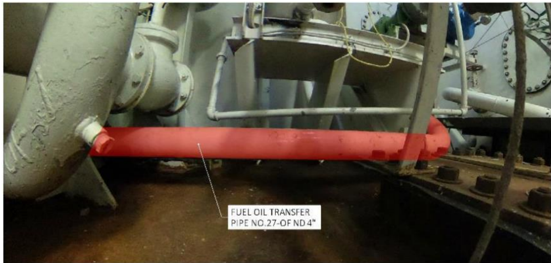
Figure 17 Fuel Oil transfer 27-OF, connection at bulkhead 138
