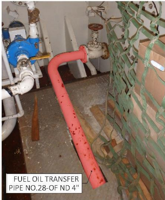
Figure 15 Fuel oil transfer, connection at bulkhead 146
