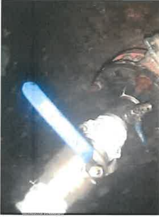
Flange fitted with a blanking valve
