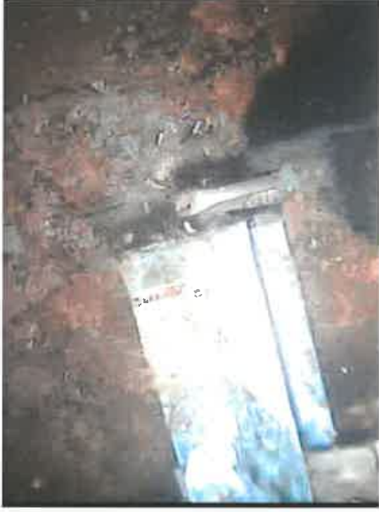
Valve with missing handle
