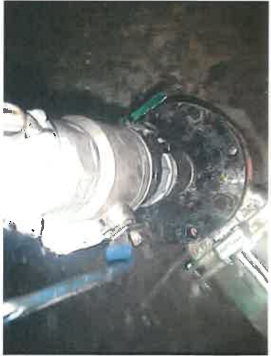
Suction hose valve fitted while pumping
