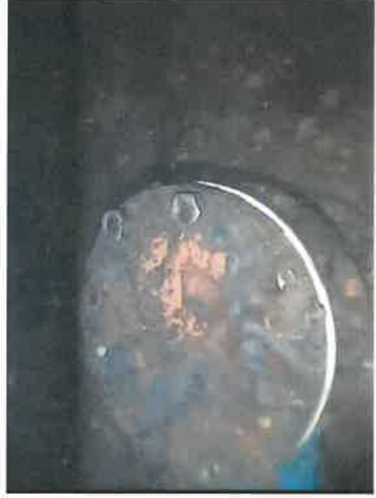
Newly applied epoxy to a small hole Tank valve caps re installed
