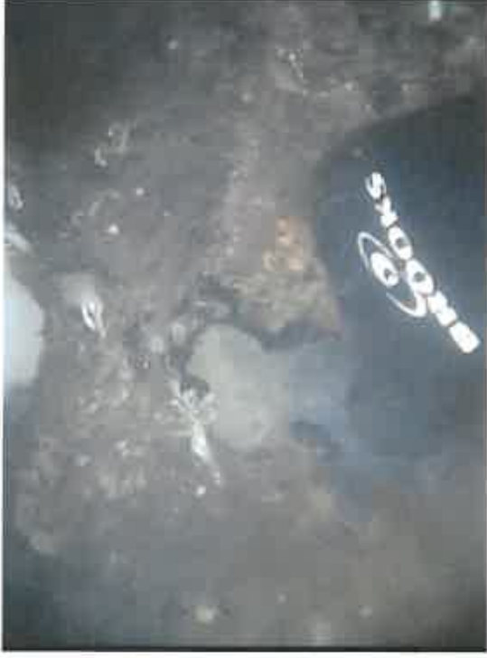
Newly applied epoxy to a small hole Tank valve caps re installed
