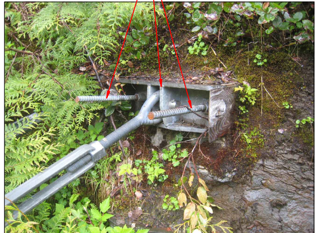
EXIST. BRIDGE MAIN CABLE END CONNECTION
