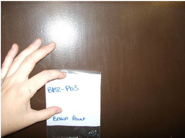
Photograph 35: Buoy Maintenance Building – Lead-Based Brown Exterior Paint
