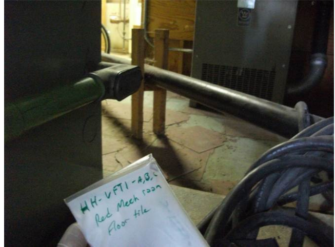
Photograph 22: Helicopter Hangar Building – ACM (VFT1) 12" X 12" Red Vinyl Floor Tile
