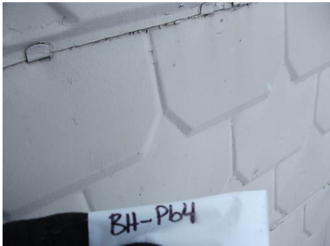
Photograph 31: Boat House Building – Lead-Based Beige Exterior Wall
