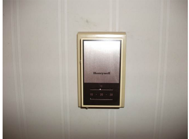
Photograph 38: Typical Mercury Containing Thermostat Observed in Buildings at CCGB Prescott
