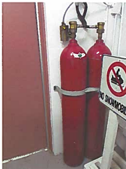
Photo 15: CO2 fire suppression system tanks.
