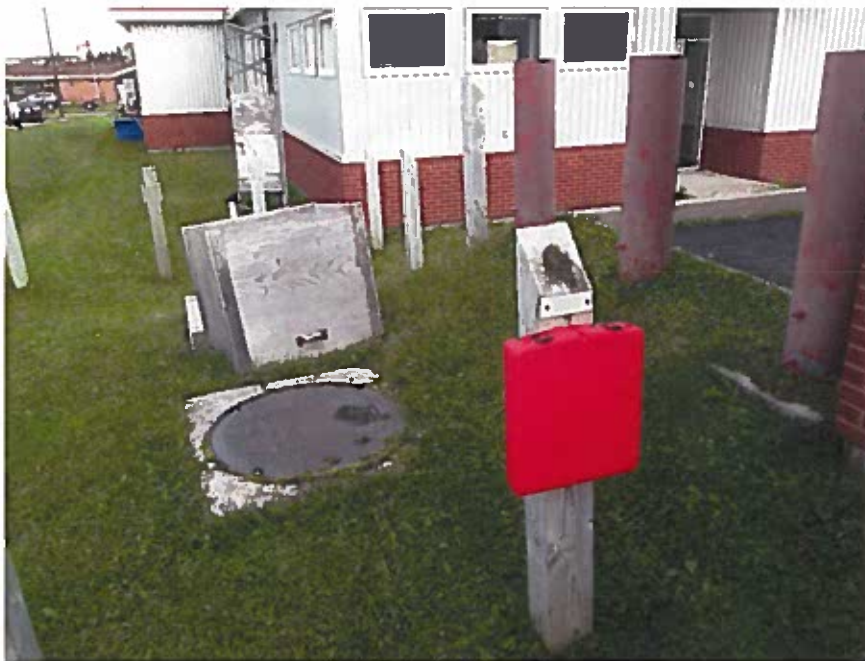
Photo 14: Filling cap and access to 4540 L UST.
