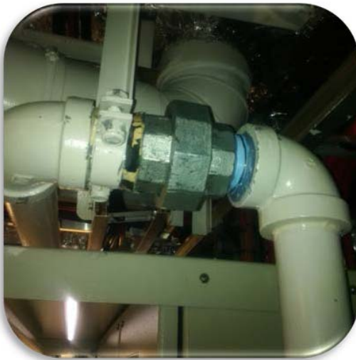
Figure 8 Nipple removed and short union installed
