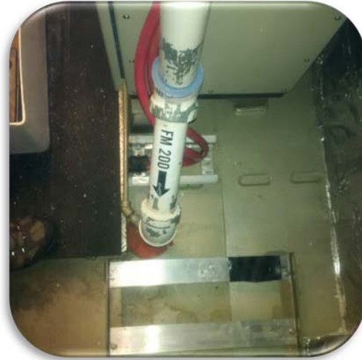
Figure 7 FM200 piping rotated inward after union modification
