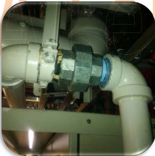
Figure 8 Nipple removed and short union installed
