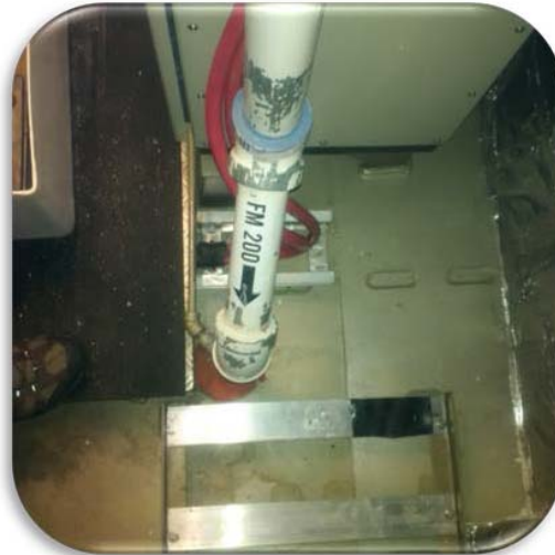
Figure 7 FM200 piping rotated inward after union modification
