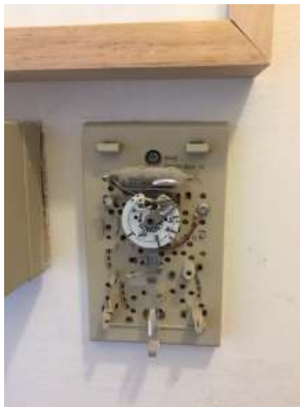
Mercury containing thermostats identified on the main floor of the property
