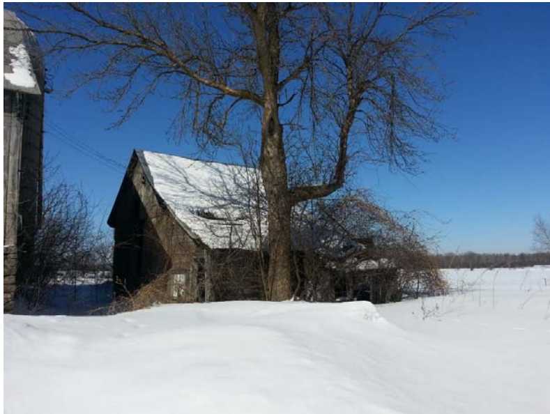
Photo 4: View of shed (building asset 97516).
