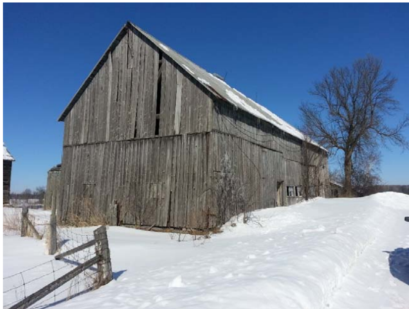
Photo 2: View of barn (building asset 97514).
