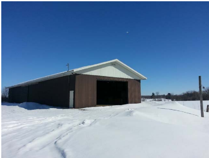
Photo 5: View of storage shed (building asset 3347).
