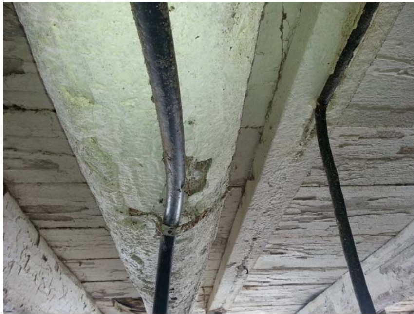
Photo 9: View of representative plaster in building 97514. Sample set PLA-01A-C.
