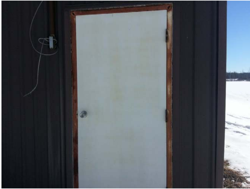
Photo 11: View of lead containing white door paint (P-05) and potential lead containing red wall paint (P-04).
