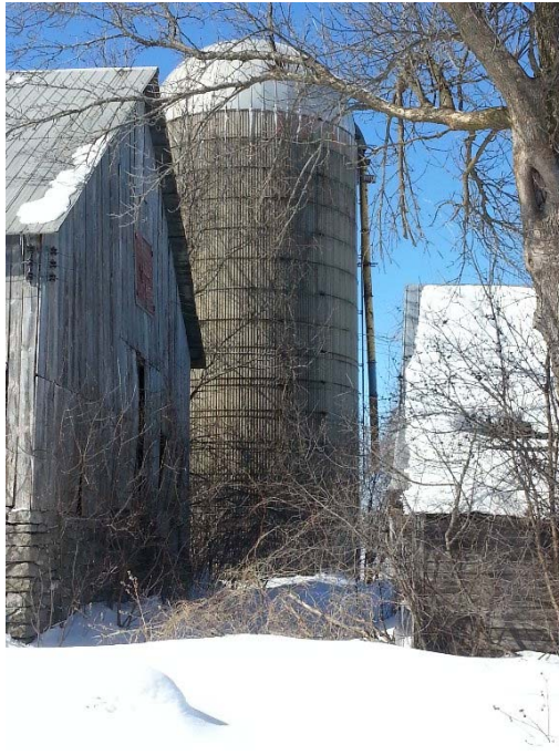
Photo 3: View of silo (building asset 3349).
