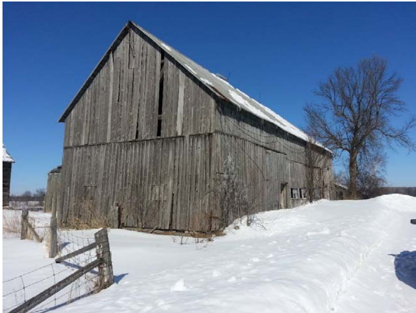
Photo 2: View of barn (building asset 97514).
