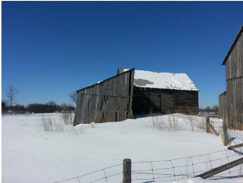
Photo 1: View of barn (building asset 3348).
