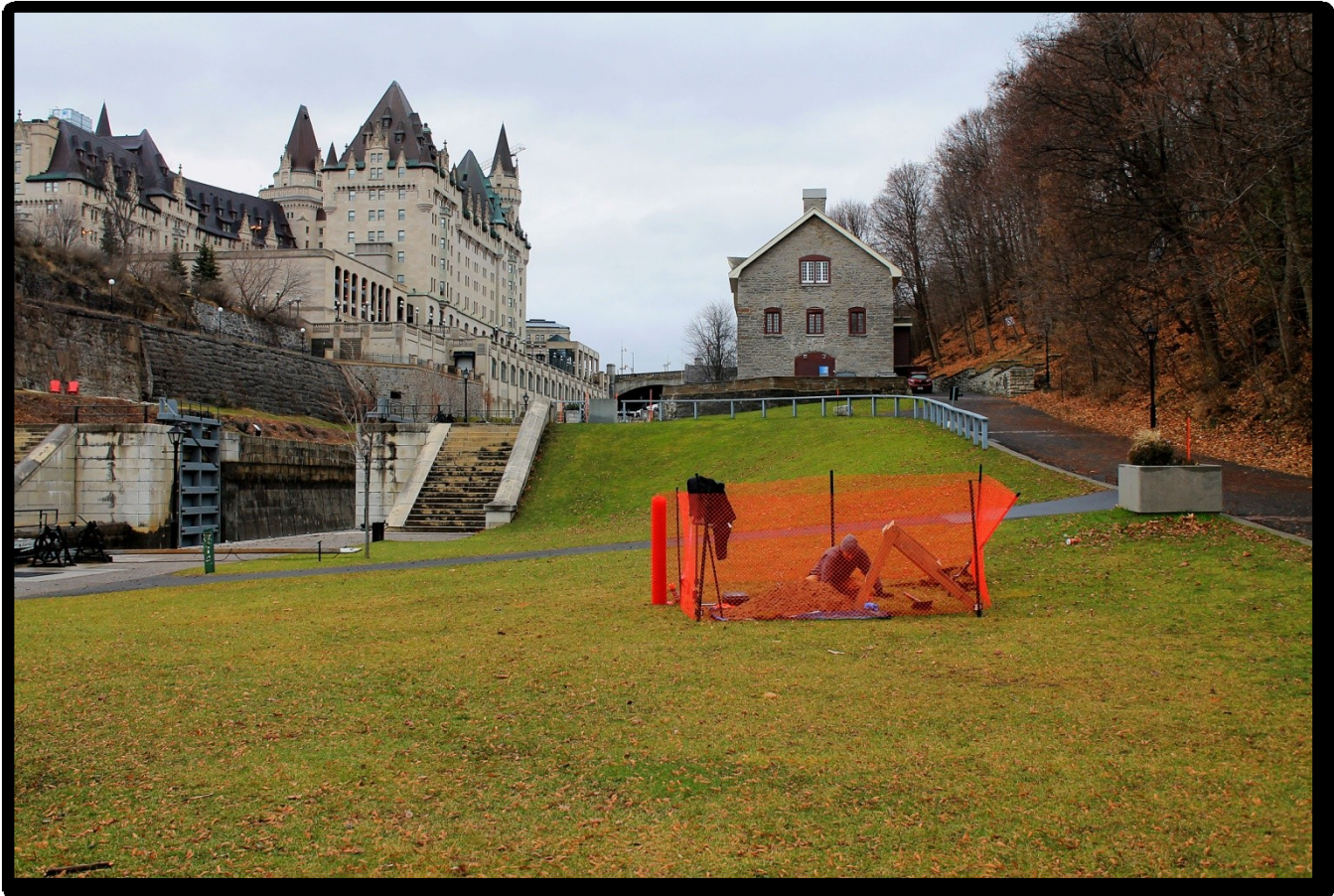
Figure 1: Excavating 34H56A at Ottawa Locks (34H99E).
