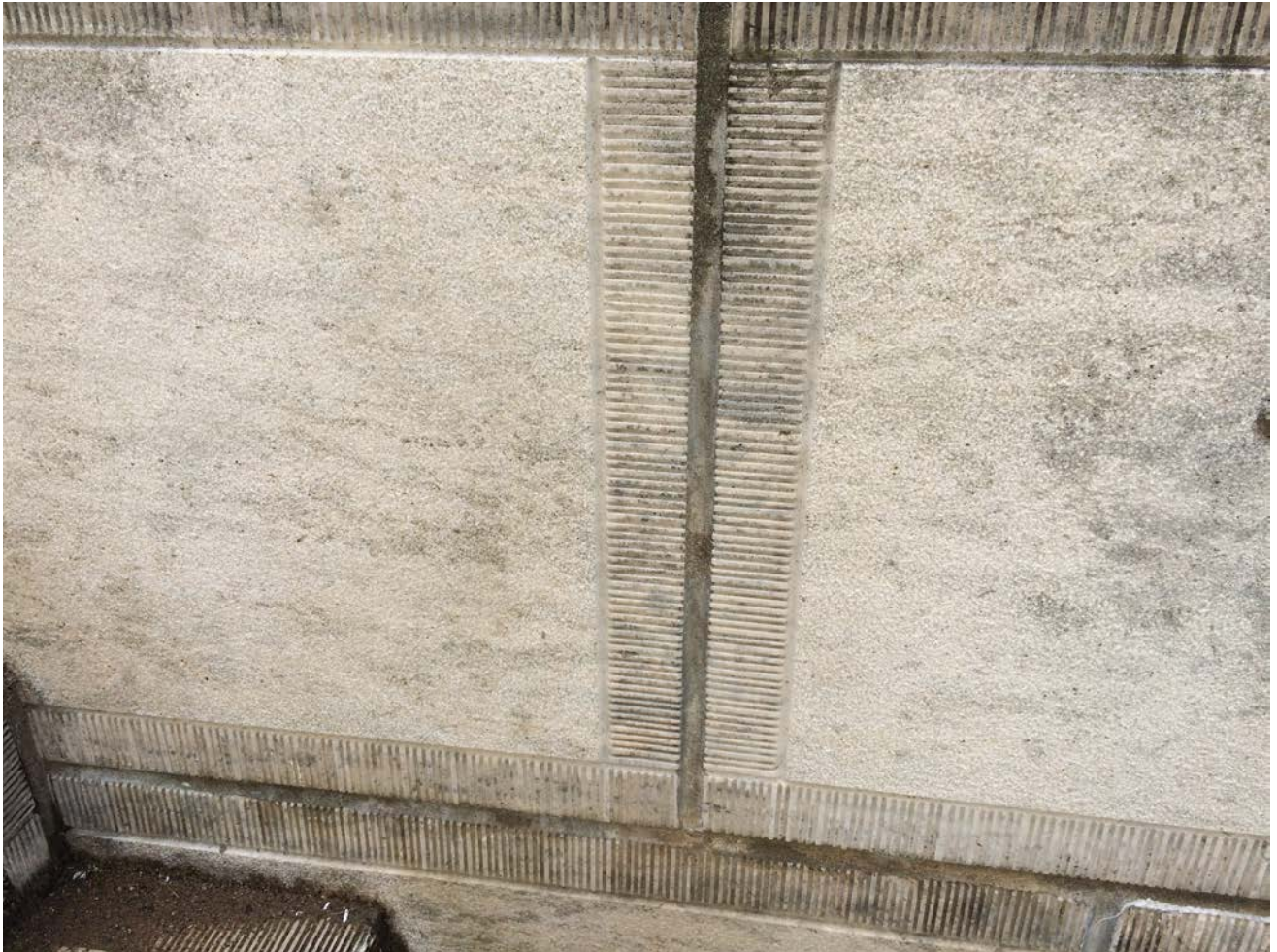
Image 1.1: Sandblasted and Dressed Block
