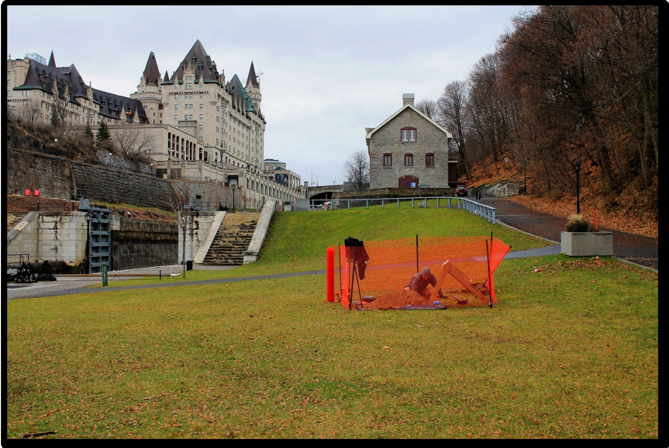
Figure 1: Excavating 34H56A at Ottawa Locks (34H99E).
