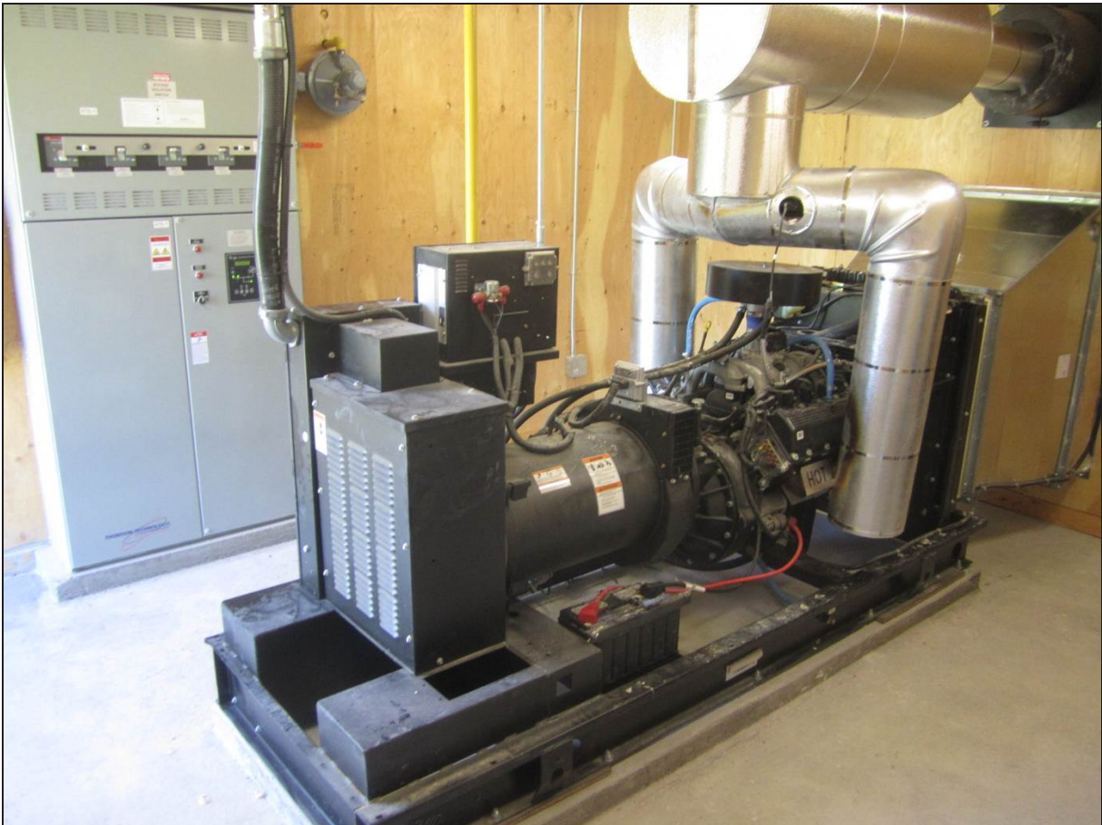
Figure 3: Natural gas generator at Timiskaming dam (installed 2012).
