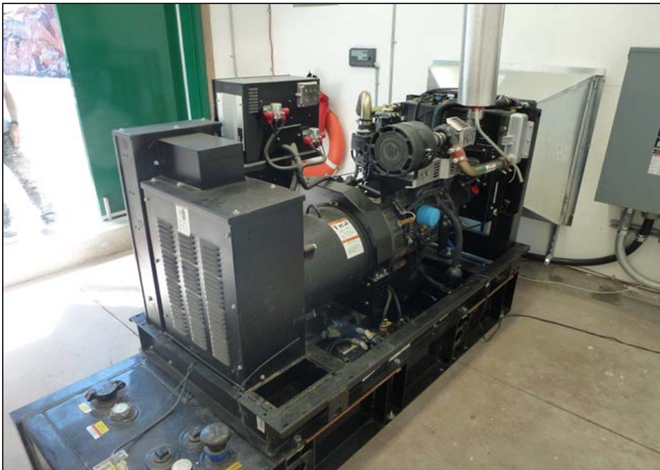
Figure 7: Diesel generator at Big Chaudière Dam.
