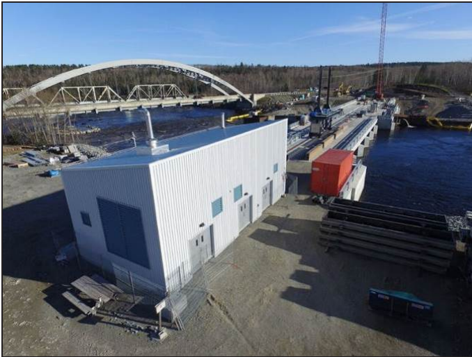
Figure 4: Service building at Latchford Dam. The generator is in the room closes to the foreground; the middle room is the main electrical room.
