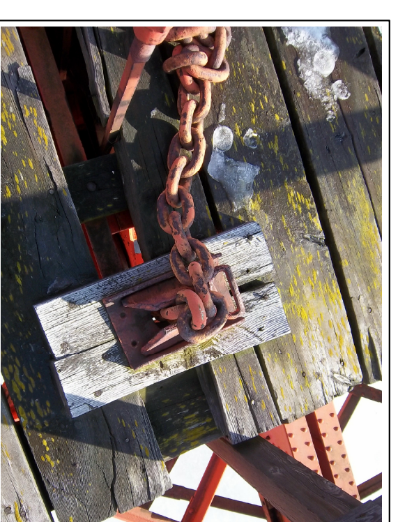
4 REPLACE CRUSHED STOP BLOCKS & REPLACE 6 - CAST WICKET CHAIN STOPS
