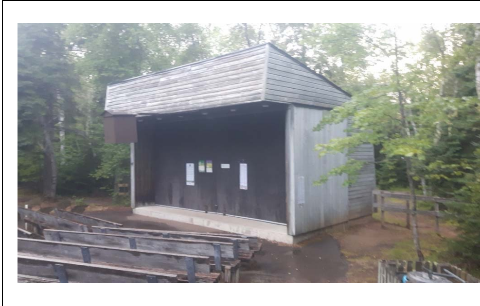
Photo 1: Outdoor Theatre, Main Theatre Building
