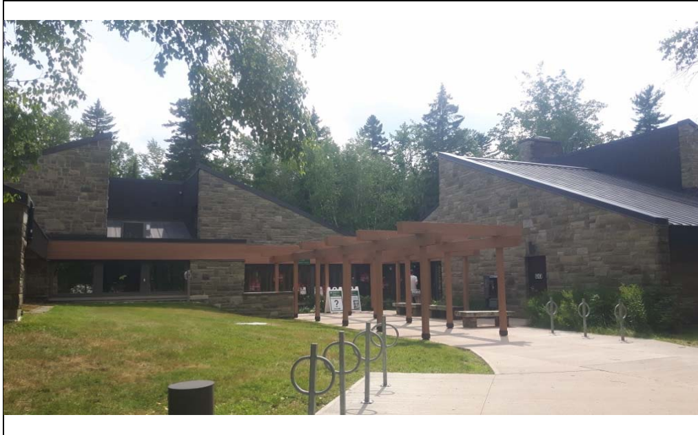
Photo 15: Administration / VRC Building
