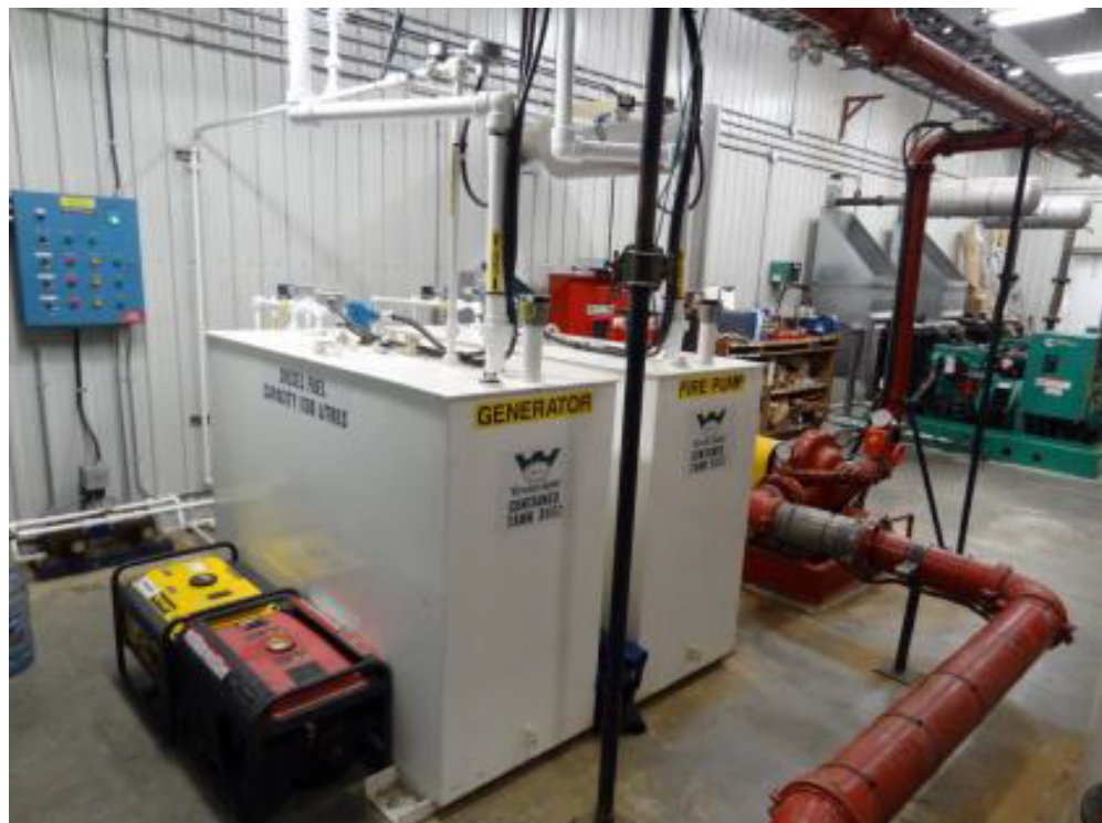
Existing Fuel Storage Day Tanks
