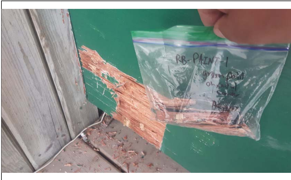
Photo 10: RB-Paint-1, Front of rental booth
