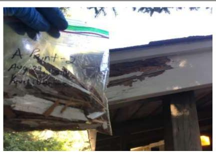
Photo 2: A-Paint-2 Roof Siding
