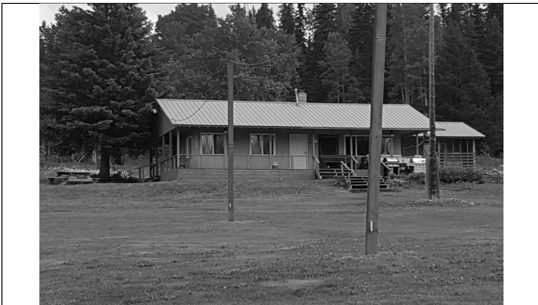
Photo 2 Date: July 13, 2017 Location: BFF Campsite - Kitchen Description: View of the building housing the kitchen, laundry and bathroom facilities.
