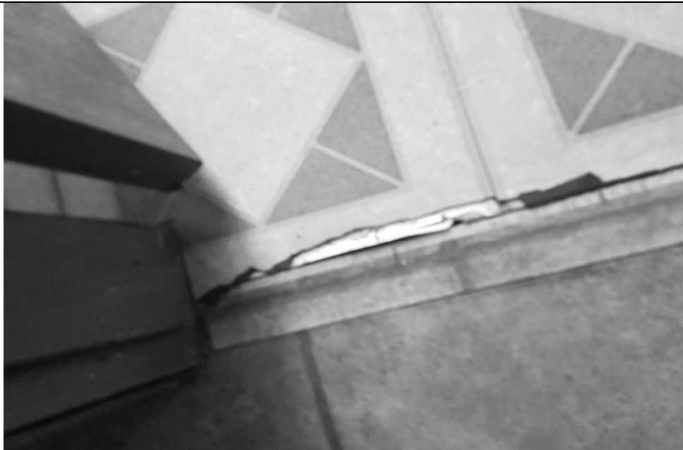
Photo 4 Date: July 13, 2017 Location: BFF Campsite - Kitchen Description: View of the built-up flooring with asbestos sheet vinyl flooring as base layer in bathroom #1.
