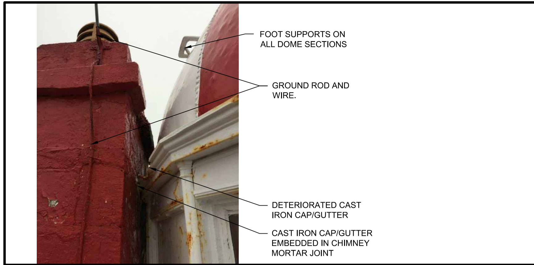
DOMES GLAZING HEAD AT CHIMNEY
