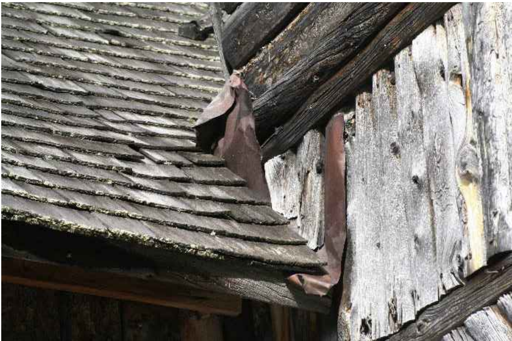
5 A-901 EXISTING STEP FLASHING SCALE
