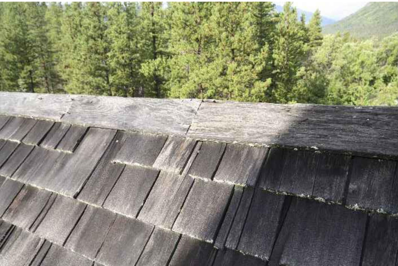
7 A-901 EXISTING RIDGE BOARDS SCALE
