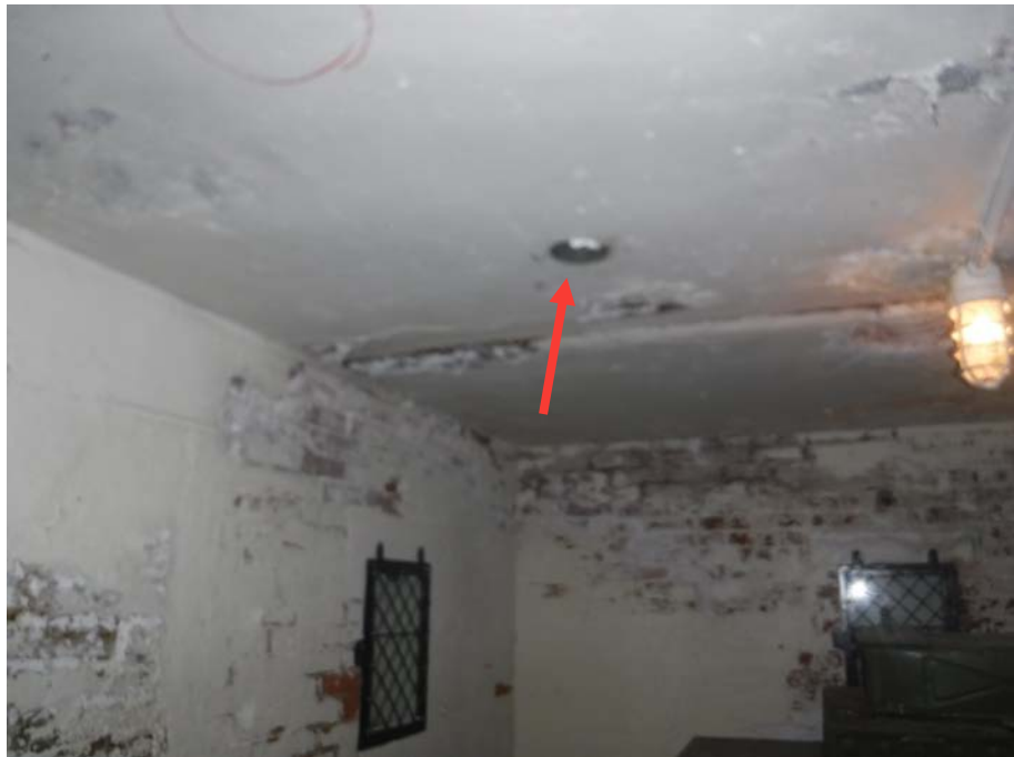
Photo 4: Underside of the "magazine" roof and core location
