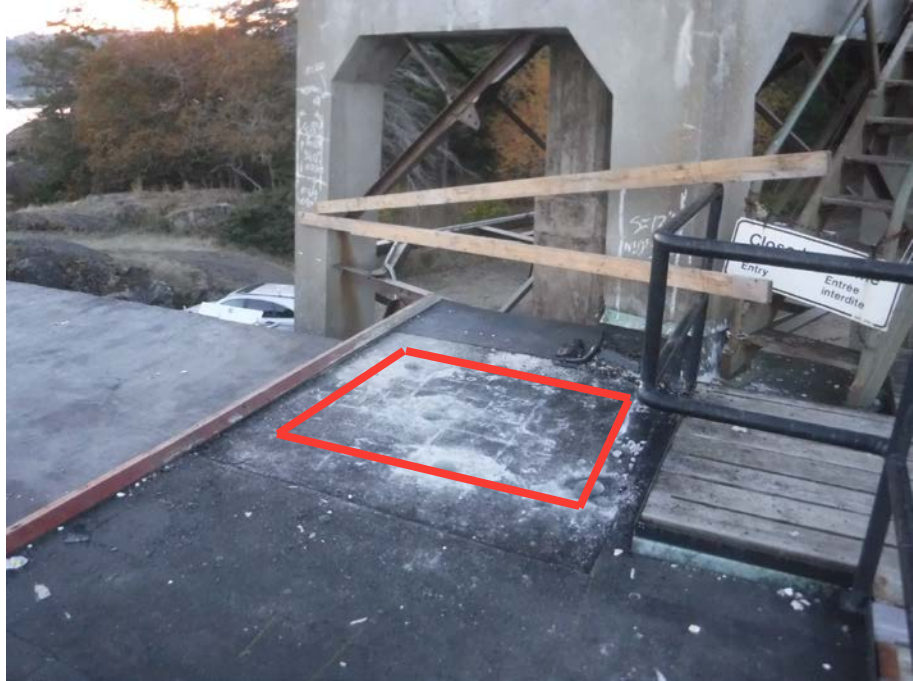
Photo 21: Roof slab top surface GPR survey area
