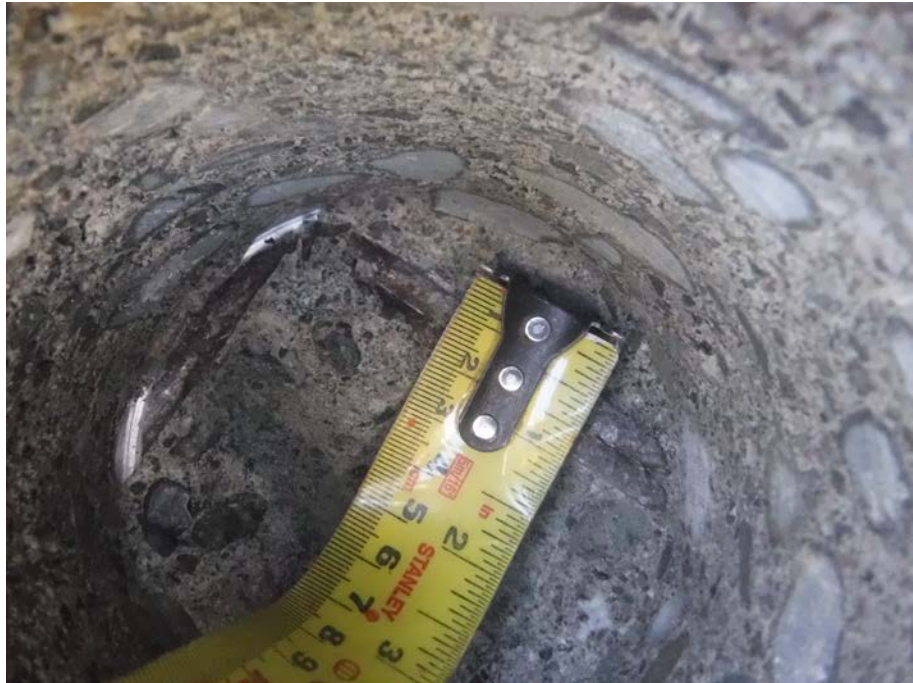
Photo 23: Steel reinforcement exposed from roof slab top surface
