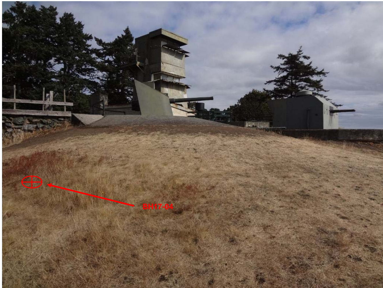
Photograph 5: Approximate location of the first borehole at the west Belmont Retaining Wall
