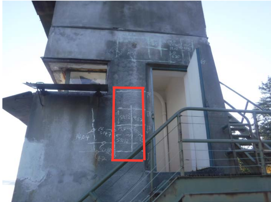
Photo 27: Area of GPR survey on wall pier
