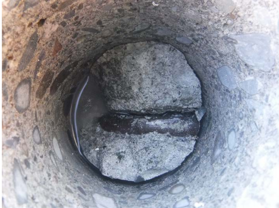
Photo 25: Bent bar cut at the upper end
