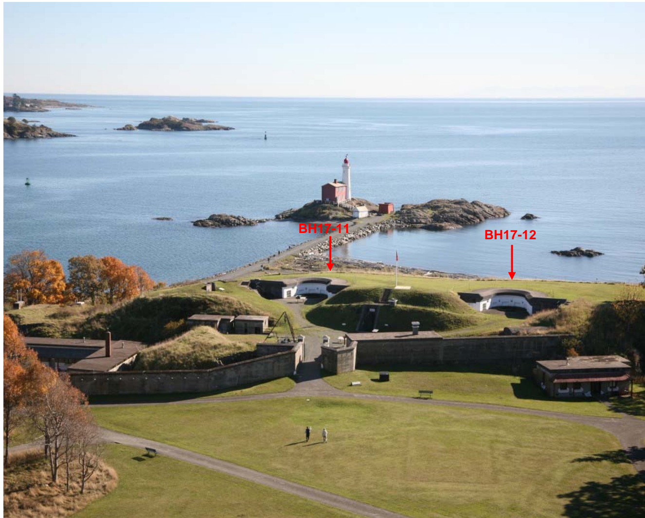
Photograph 15: Approximate locations of boreholes at the Lower Battery Underground Magazine
