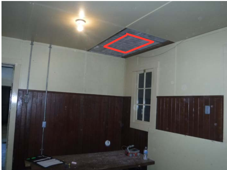
Photo 22: Roof slab soffit GPR survey area
