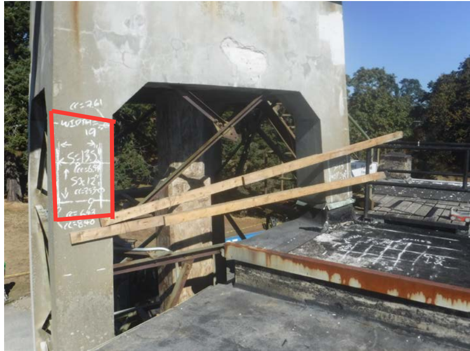
Photo 17: GPR survey on the south face of the southwest leg
