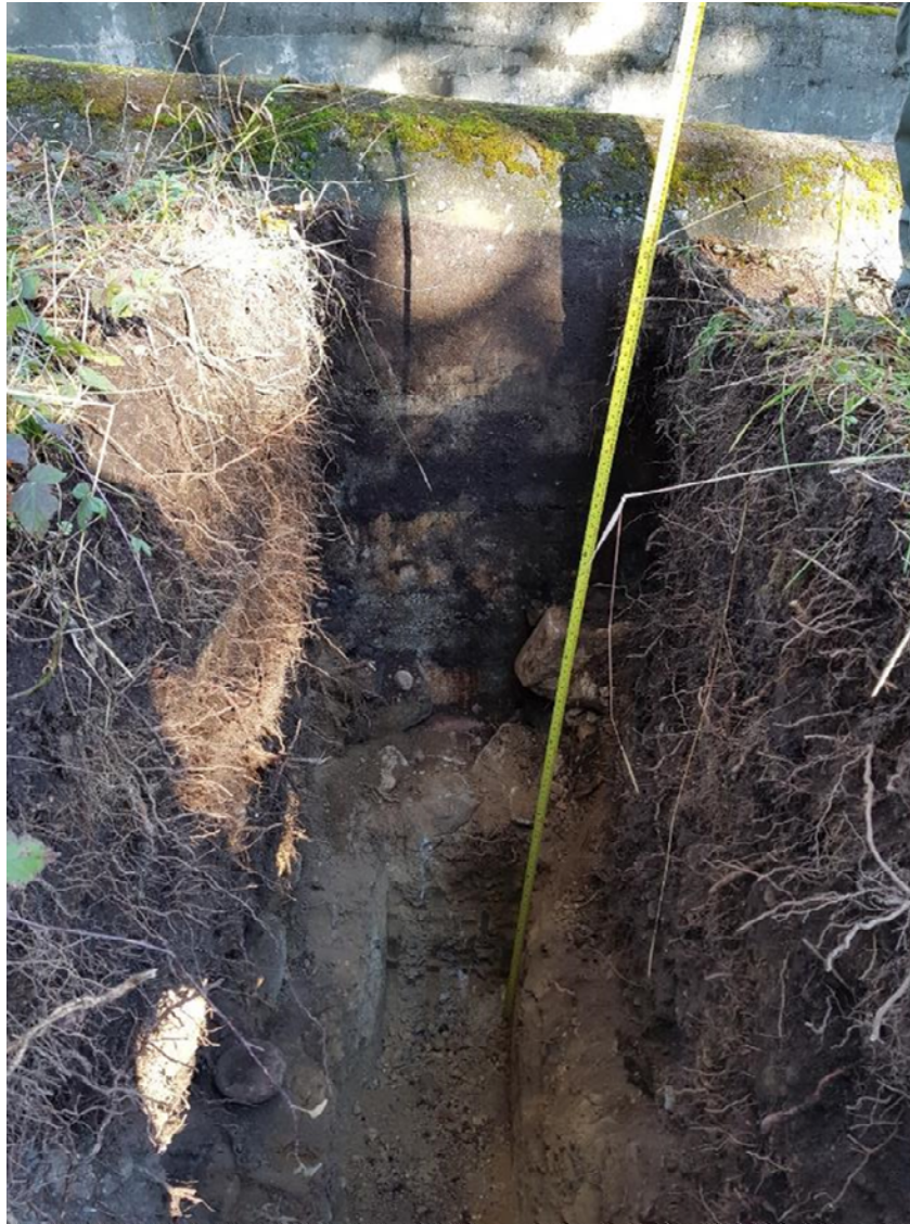
Photograph 10: Test pit at the south Searchlight Engine Room Retaining Wall (TP17-01)
