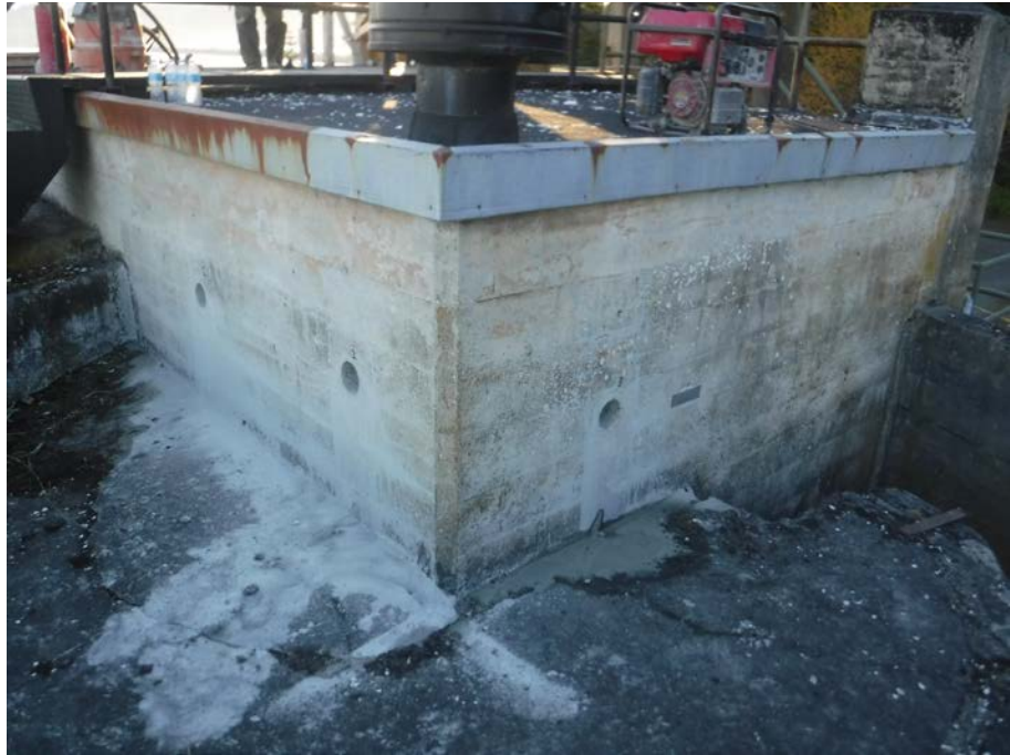
Photo 1: Locations of core samples from the exterior walls
