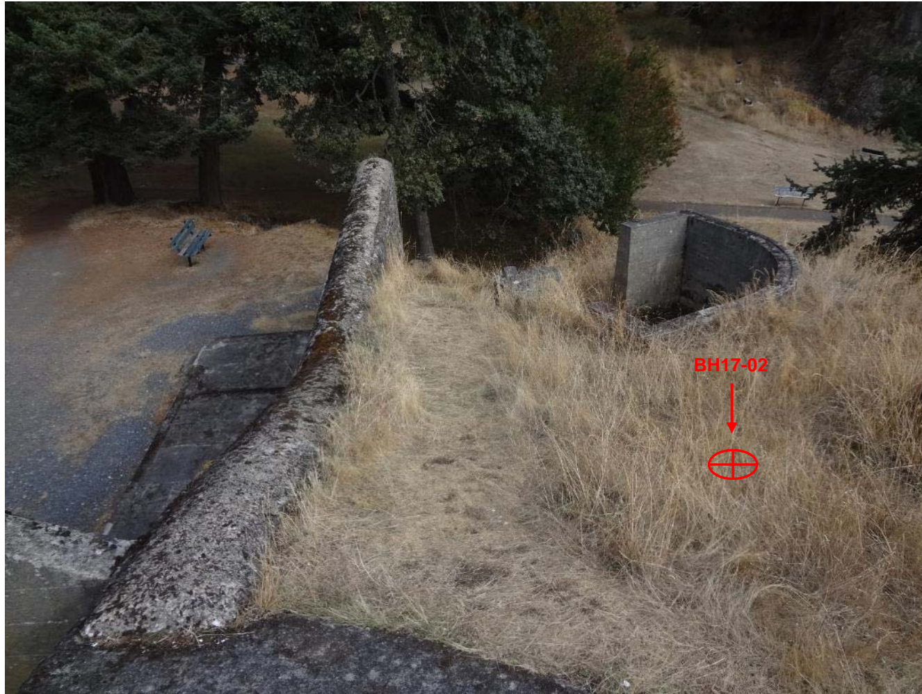
Photograph 8: Approximate location of borehole at the east Belmont Retaining Wall
