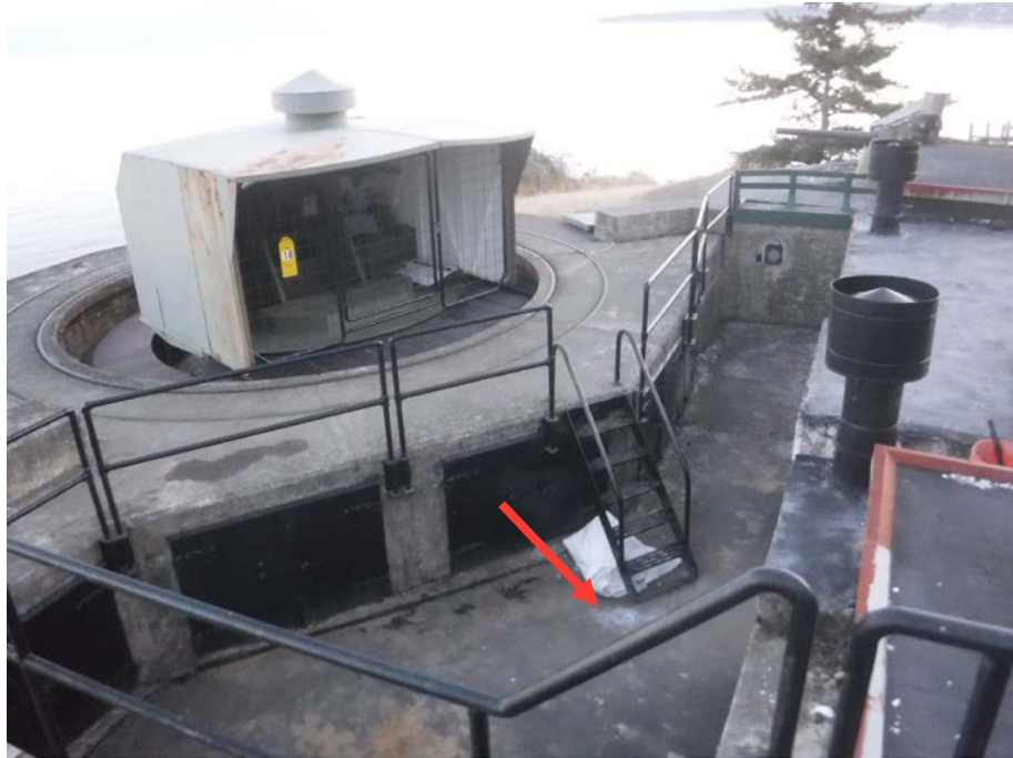
Photo 3: Location of full-thickness core from "magazine" roof
