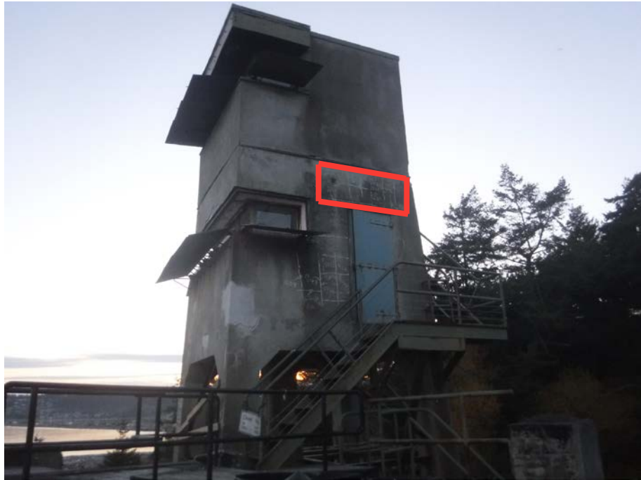
Photo 13: Director's Tower floor beam GPR survey area
