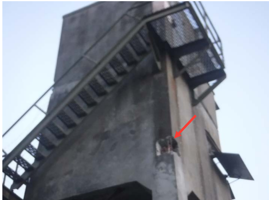
Photo 18: Location of reinforcement size review on the northwest leg
