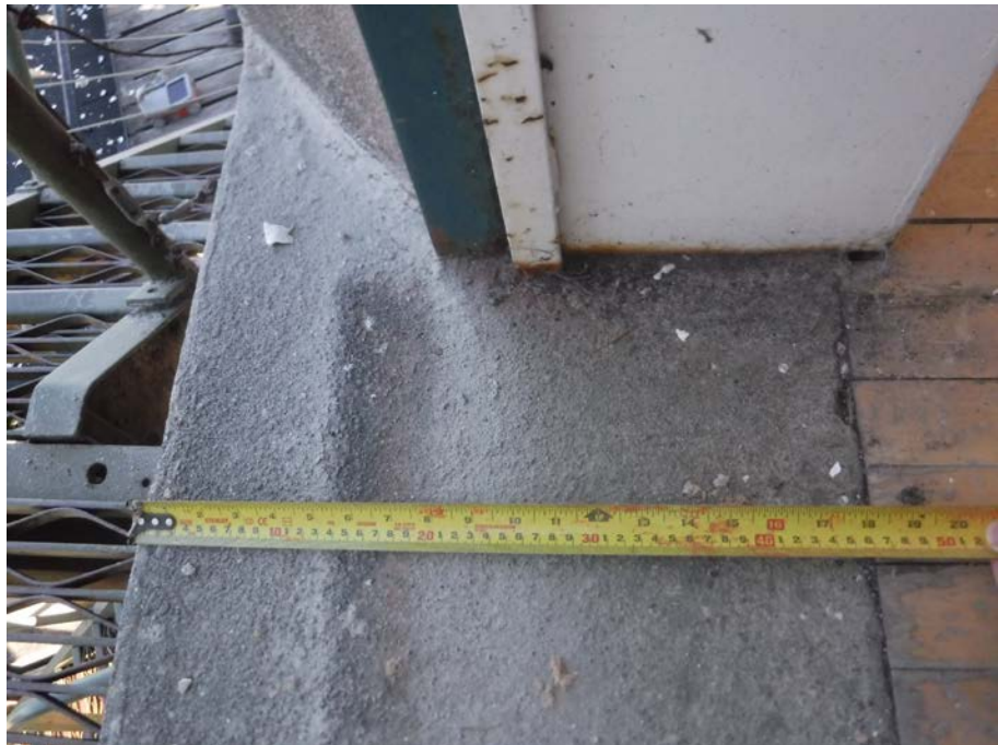
Photo 26: Wall pier thickness measured at door opening
