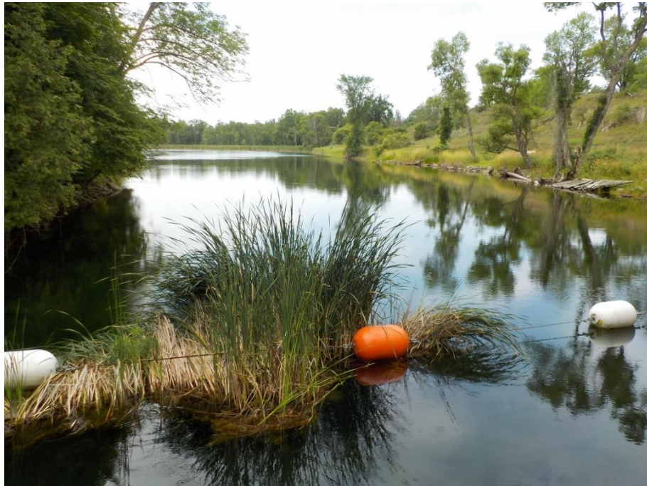
Photo #3 View of Tay River and Bobs Lake upstream from the existing dam Bobs Lake Dam Tay Valley Township (Ontario)
