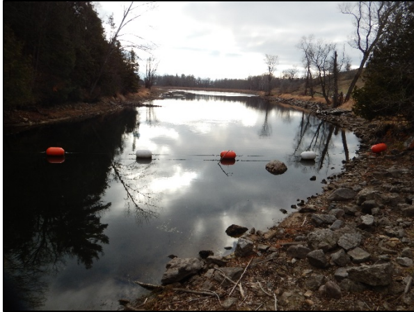
Photo 11 (left): Outlet bay in Bobs Lake from the north bank at the dam.
