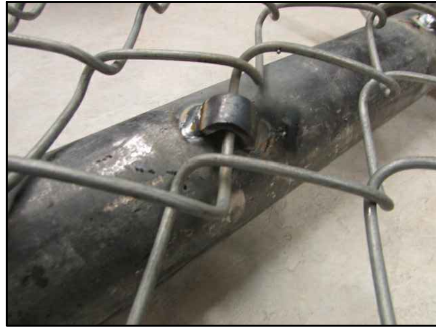
4 CHAIN LINK FENCE FABRIC CURVED GALVANIZED STEEL CLIPS A2.3 SCALE - 1:25
