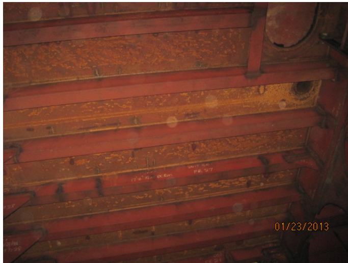
4.35: F.O. Deep Tank Starboard - Longitudinal Bhd
