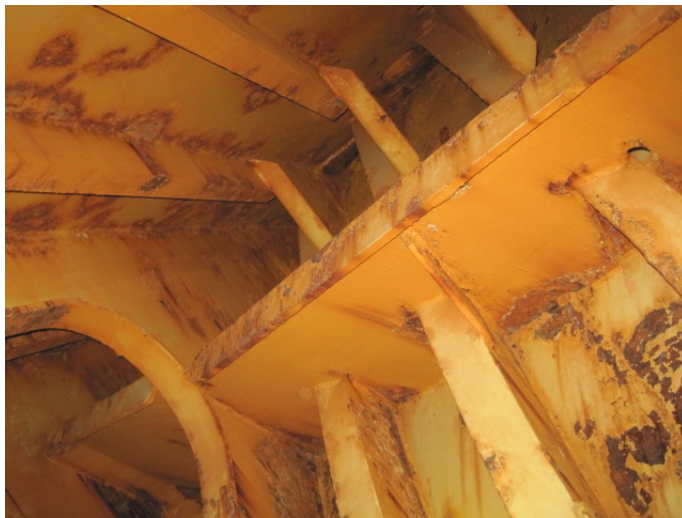
4.14: Aft Trimming Tank - Deck and Side Shell
