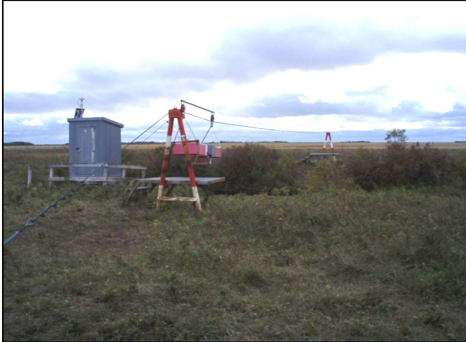
Photograph 1: Typical cableway and towers.
