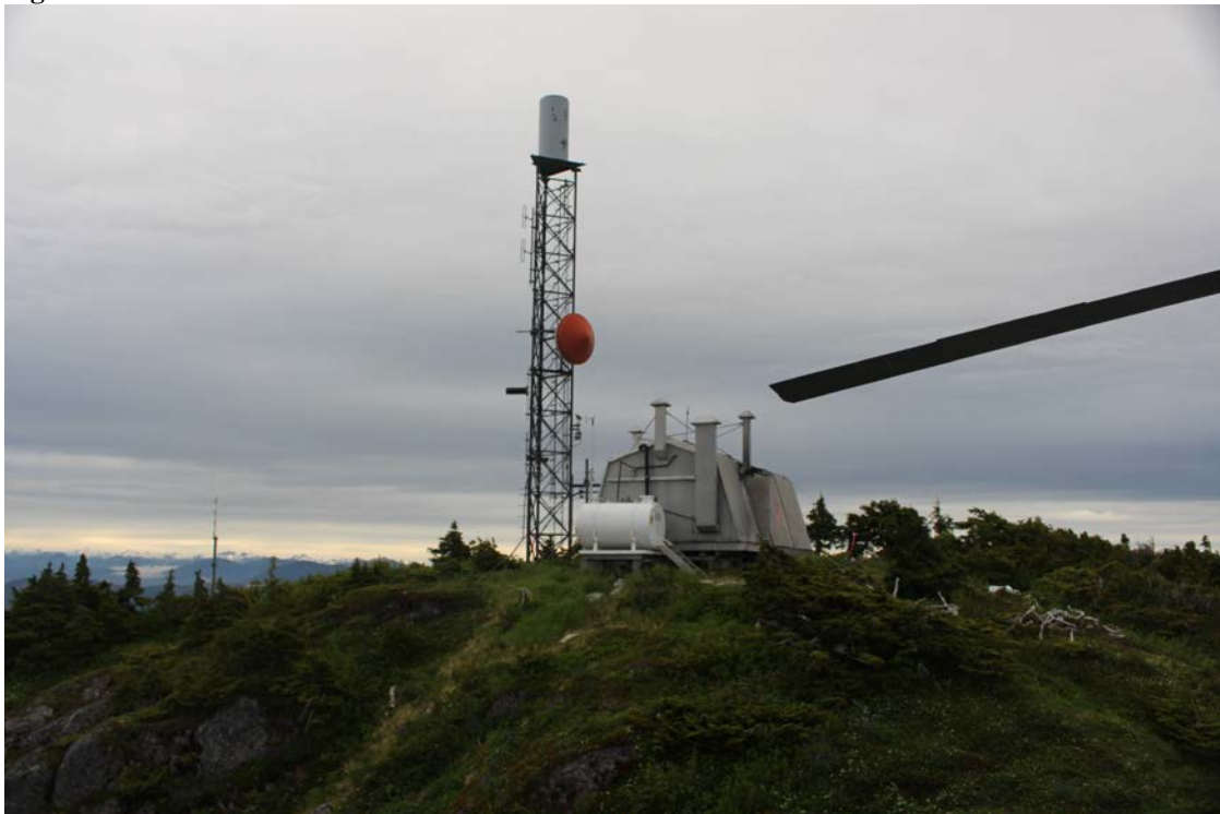
Figure 4 - Existing Tower and Building
