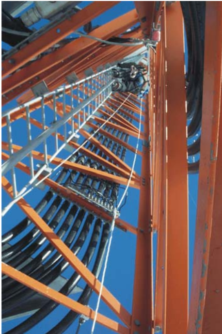
Figure 2-6 TGBs are installed near the cable bridge entrance where the transmission lines leave the tower for their horizontal run across the cable bridge into the communication room. Figure 2-7 The TGB has to be mounted below the cable grounding kits to ensure that the discharge path of a potential lightning strike will be downwards to the TGB where all cable grounding straps are tight together.
