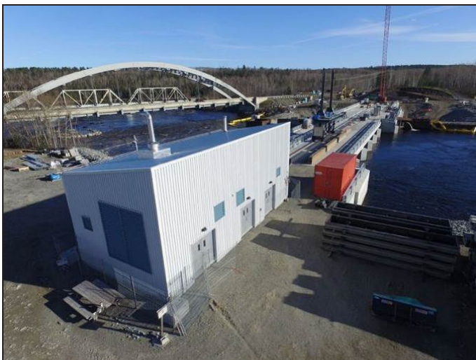
Figure 4: Service building at Latchford Dam. The generator is in the room closest to the foreground; the middle room is the main electrical room.
