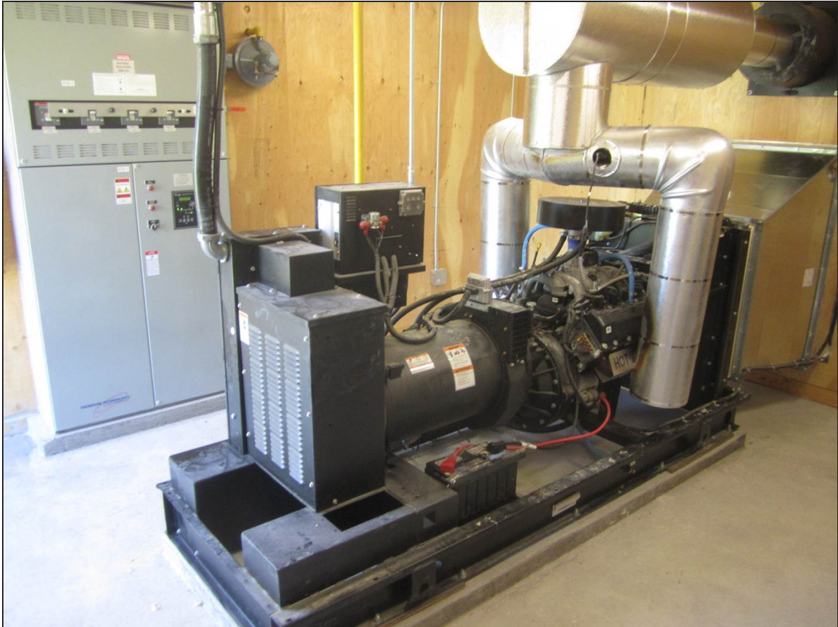
Figure 3: Natural gas generator at Timiskaming dam (installed 2012).
