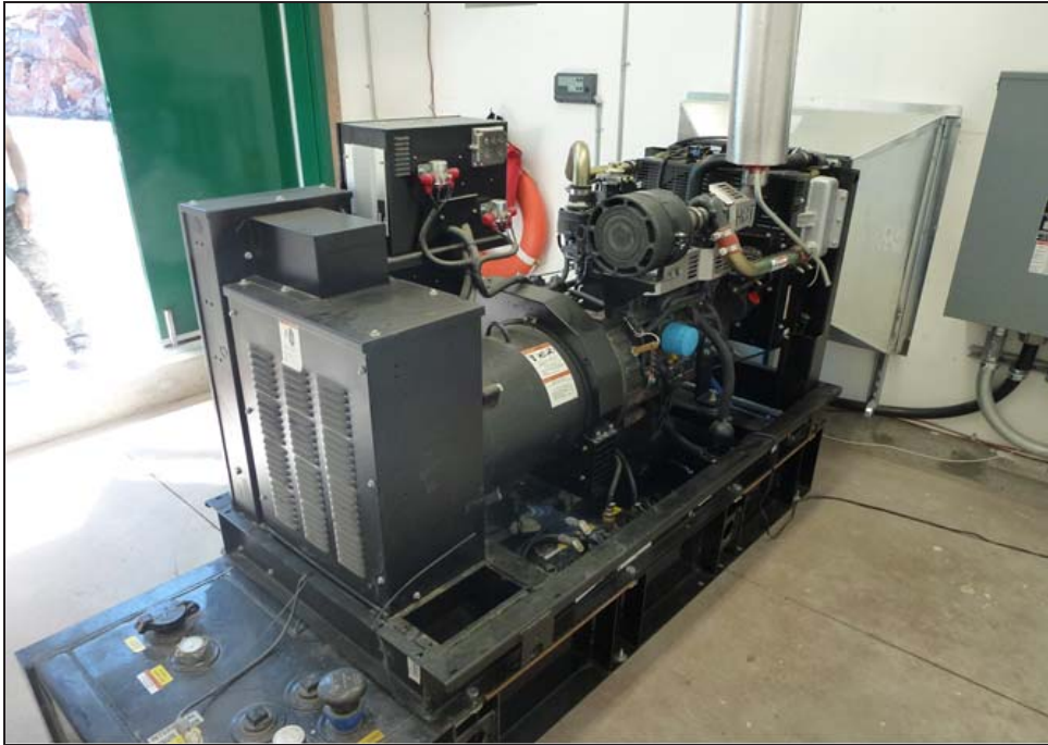
Figure 7: Diesel generator at Big Chaudière Dam.
