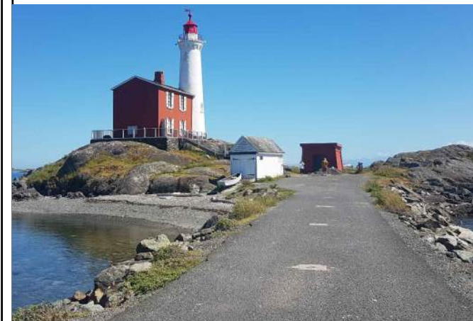
FISGARD LIGHTHOUSE WITH WASHROOM BUILDING - LOOKING SOUTH, HCS 2017
