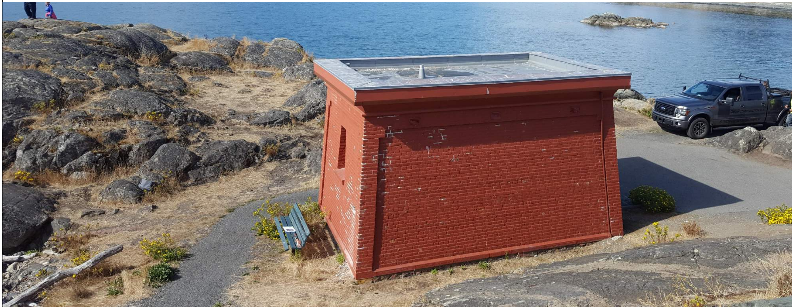
FISGARD LIGHTHOUSE WASHROOM BUILDING - LOOKING WEST
