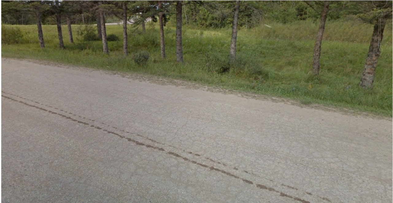
Figure 1 -Example of Alligator Cracking
