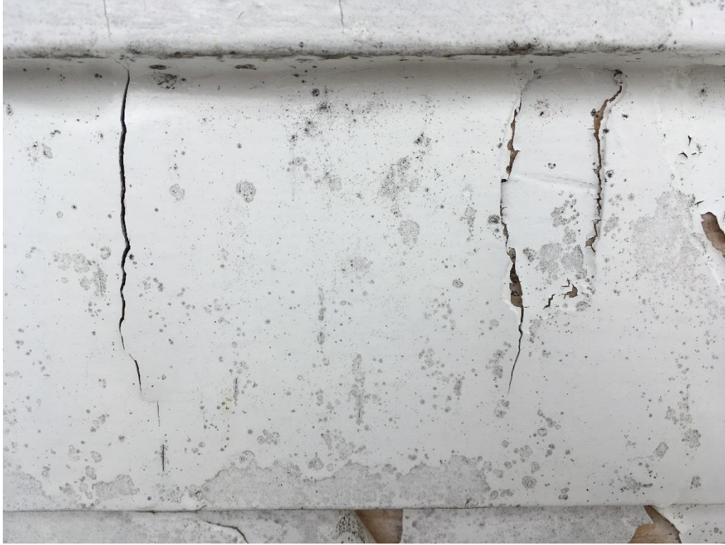
Photo 9 – Mould growth on painted clapboard – east side of building
