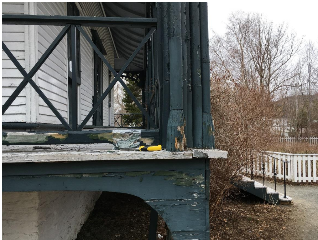
Photo 7 – Veranda section at northeast corner of building (note rot/deterioration and peeling paint) – Sample HC-P7
