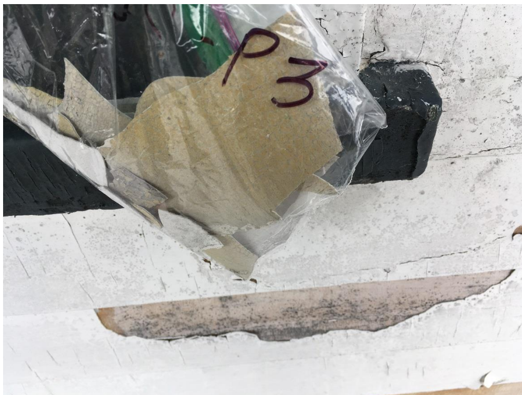
Photo 6 – Suspect mould on paint (Sample HC-P3) and on underlying clapboard
