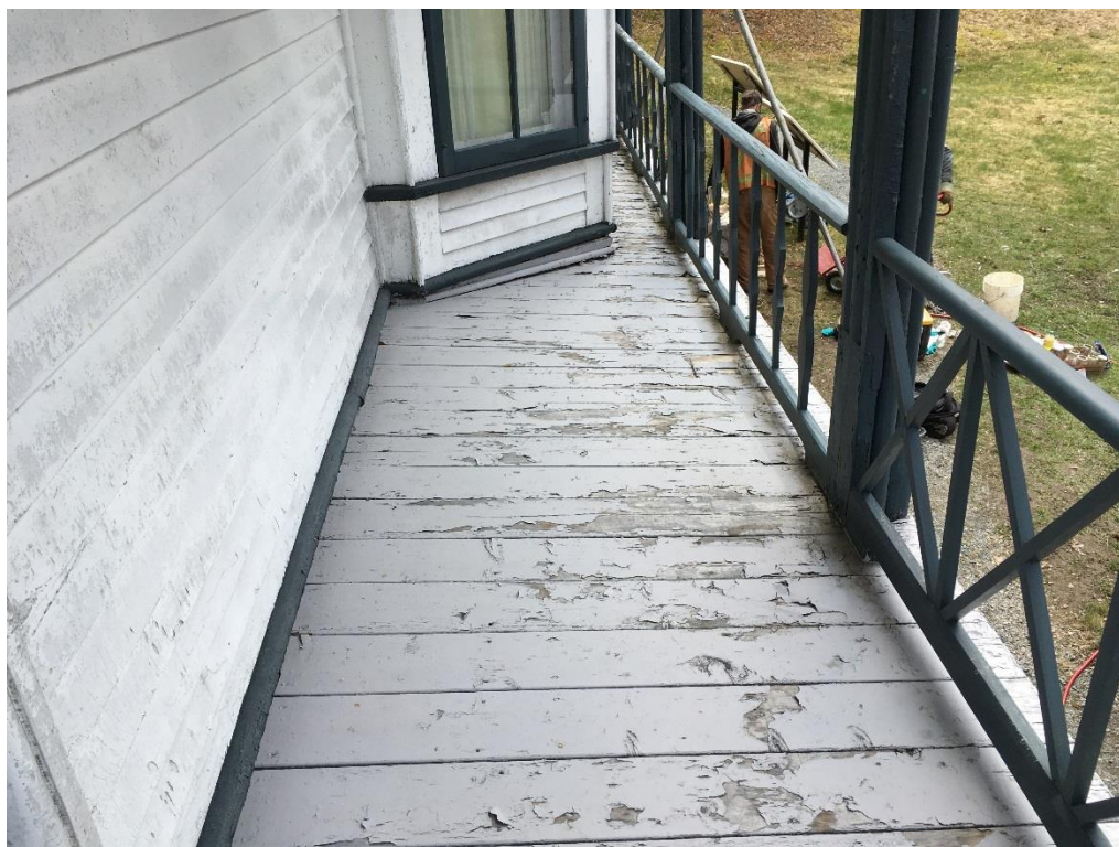
Photo 8 – Veranda deck at west side of building (note peeling/flaking paint)
