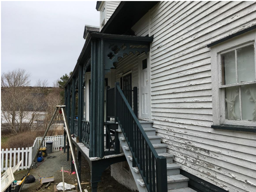
Photo 10 – Peeling paint on west side of building.
