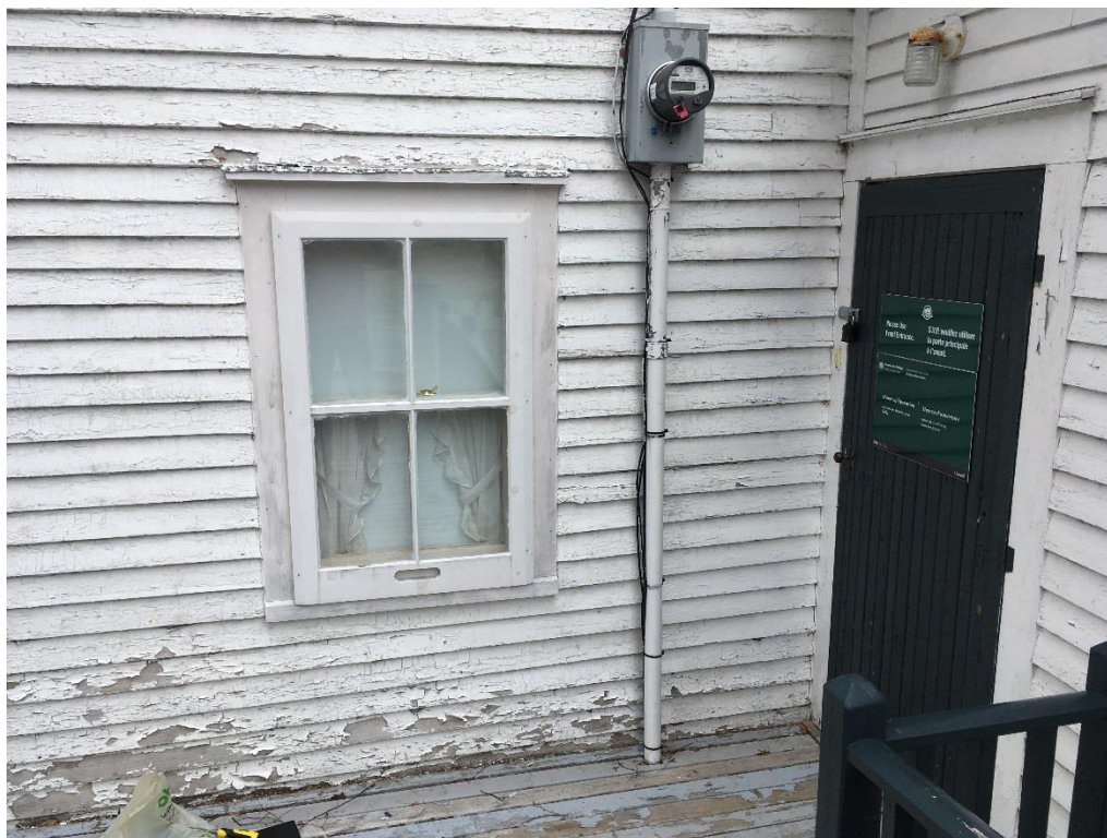
Photo 5 – South side of the building with peeling paint (Sample HC-P2 from under window)
