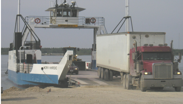
Fort Providence Ferry crossing of the Mackenzie River on Yellowknife Highway 3 near junction with Mackenzie Highway 1. A new bridge is under construction here.
