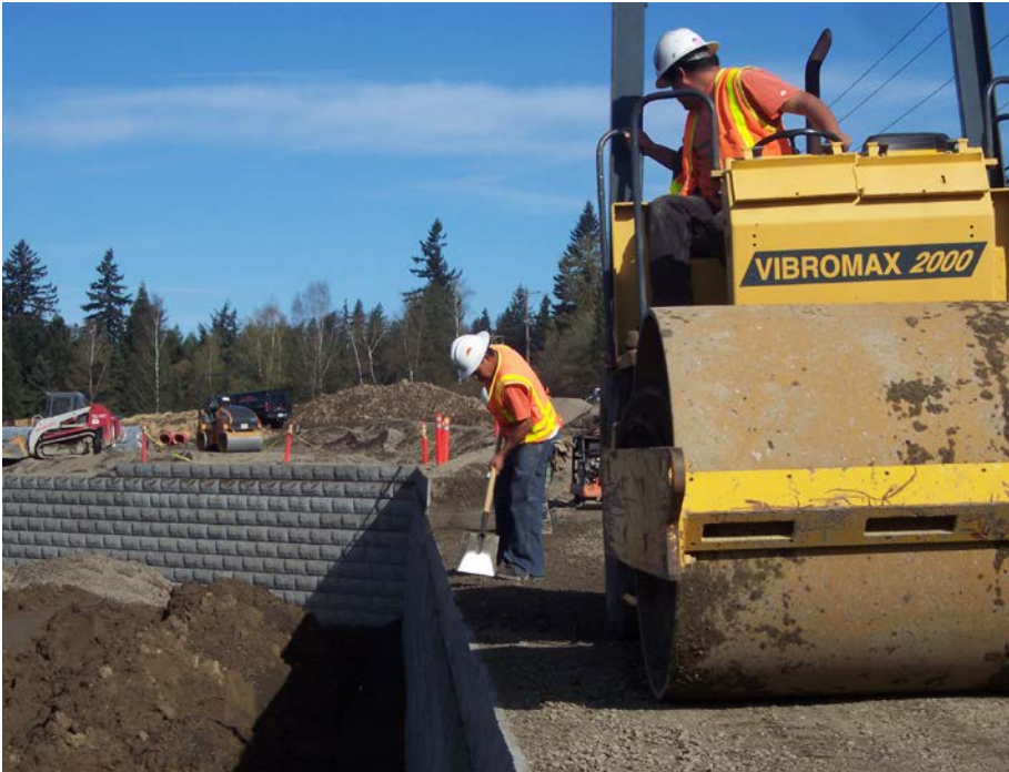
ABOVE & LEFT: THE COMPACTING OF BACKFILL
