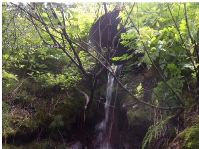
Figure 25: TCH km 28.8 (TCHGlacier_14.8) – Hanging culvert on downstream, westbound side of TCH (left) and watercourse downstream below the culvert outlet on the westbound side (right)
