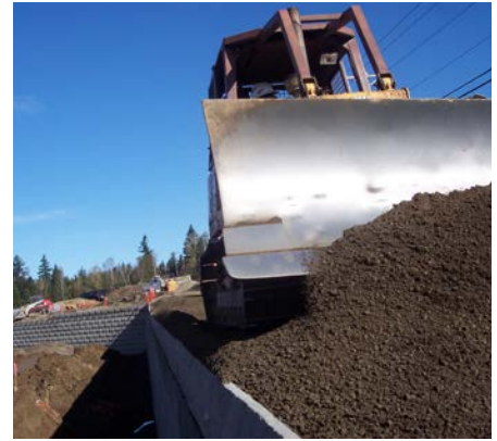
ABOVE & LEFT: THE COMPACTING OF BACKFILL
