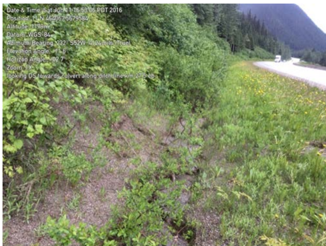
Figure 21: TCH km 27.5 (TCHGlacier_16.2) – Watercourse on upstream, eastbound side (left) and armoured section downstream below the culvert outlet on the westbound side (right)
