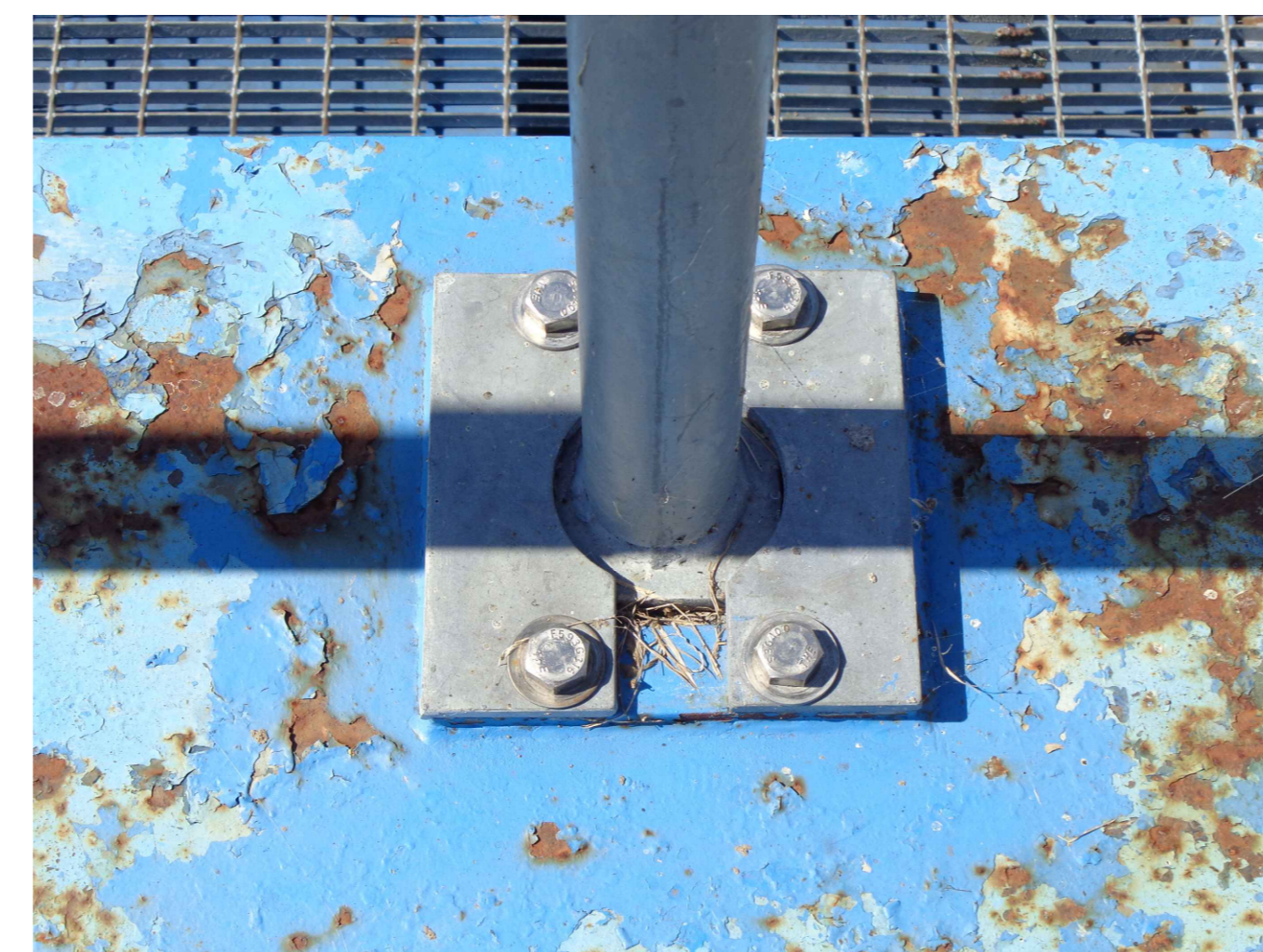
C6 ANCRAGES GARDE-CORPS GUARDRAIL ANCHORS
