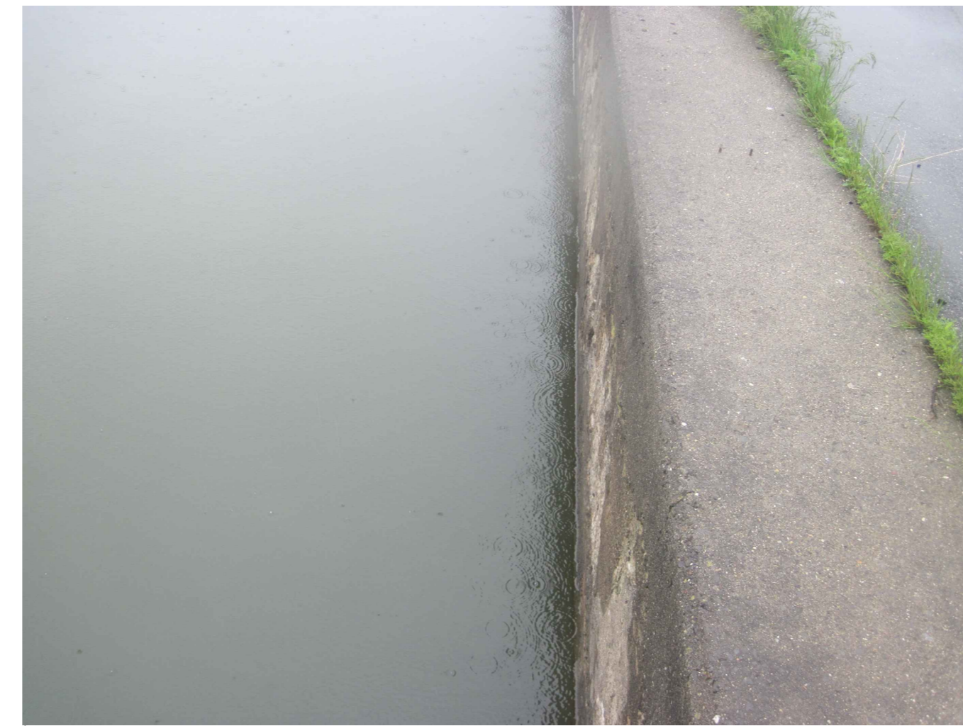
C3 MUR DU QUAI WALL OF WHARF
