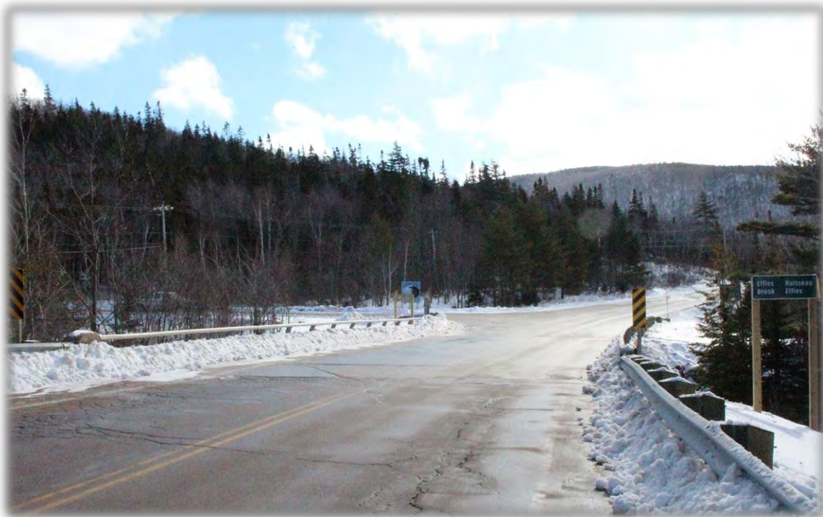
Bridge Deck (facing south)
