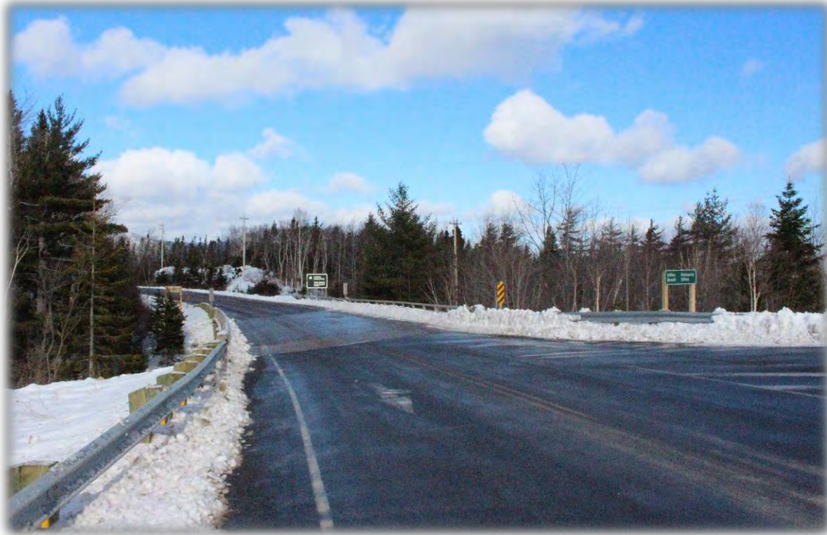
Bridge Deck (facing north)
