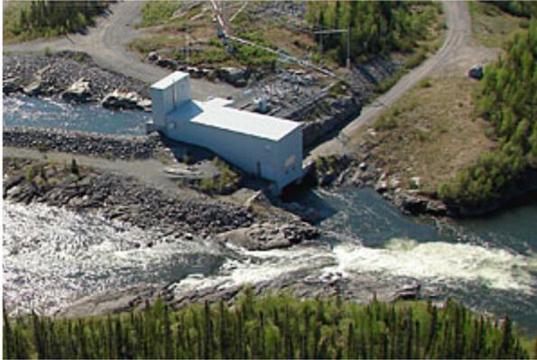
The Snare River hydro system is located some 140 km Northwest of Yellowknife in the Tlicho First Nations territory. It consists of five hydroelectric facilities generating 28 MW now serving the City of Yellowknife, and the municipalities of Behcho Ko and Dettah.
