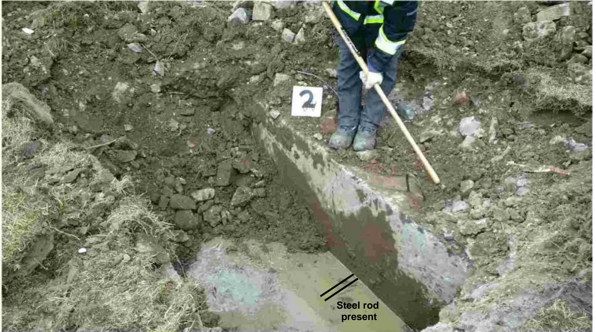
Photo 2 – Test pit TR-02 – Concrete installation with steel rod
