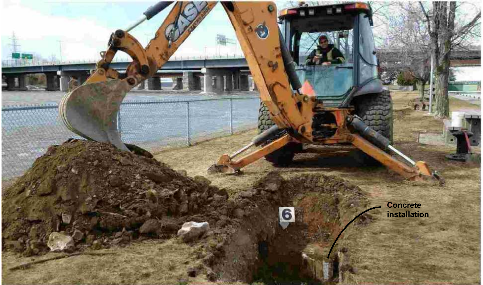
Photo 6 – Test pit TR-06 – Concrete installation
