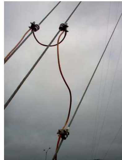
Figure 2-2 Individual grounding of guy cables near anchors above the preformed guy grips using stainless steel ice breakers. Figure 2-3 Ice breakers are mounted above preformed guy grips, preventing ice from pushing down on guy cable out from guy grip. This also provides a corrosion resistant bond of the stranded copper ground cable via stainless steel plates to the hot-dipped galvanized guy cables.
