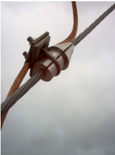
Figure 2-2 Individual grounding of guy cables near anchors above the preformed guy grips using stainless steel ice breakers. Figure 2-3 Ice breakers are mounted above preformed guy grips, preventing ice from pushing down on guy cable out from guy grip. This also provides a corrosion resistant bond of the stranded copper ground cable via stainless steel plates to the hot-dipped galvanized guy cables.
