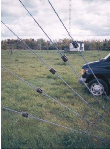
Figure 2-4 shows part of the base section of an old 220 feet (67 m) isolated tower sitting on top of the insulator. The spark gap arrester has to have its contact balls positioned horizontally to prevent water from shortening the gap. Figure 2-5 shows isolated guys.
