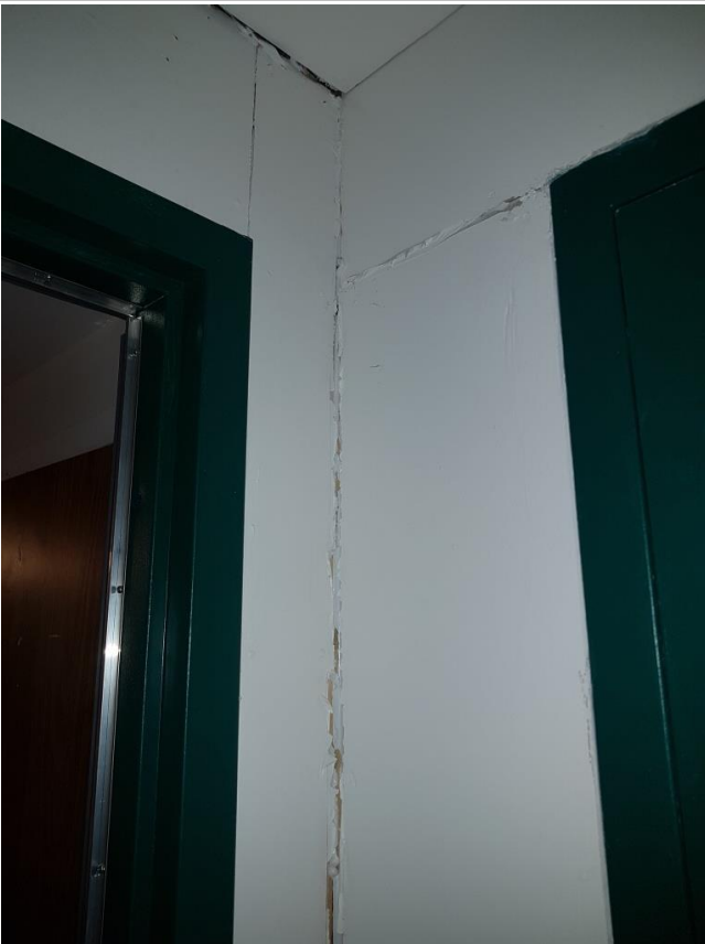
Photo 25 – Trailer, Separation at Porch/Trailer Walls and Ceiling
