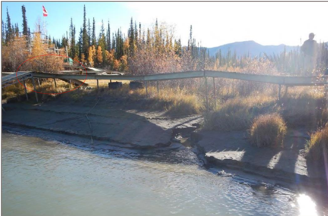
Photo 4: Existing dock at a typical seasonal low water level. New dock design is for the dock #1 on-shore grillage anchor to be located just behind the existing fixed dock to the left of the ramp (circled). Photo taken September 20, 2016
