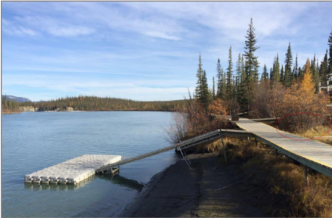
Photo 5: Existing dock at a typical seasonal low water level. New dock design is for the dock #1 on-shore anchor grillage and gangway ramp abutment to be located just behind the existing fixed dock (circled). Photo taken September 20, 2016
