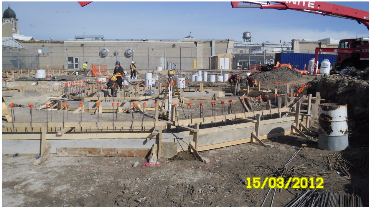
Photograph 1: Facing North from south side of building, formed footing foundation on bedrock.
