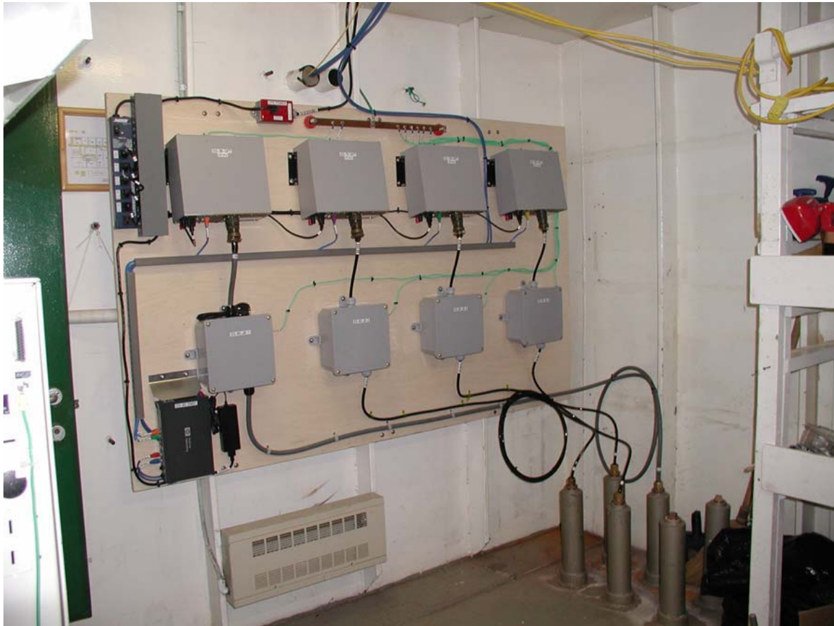
Photo 1. GPT units, junction boxes (under GPTs), transducer conduits, and transducer cables between junction boxes and conduits.
