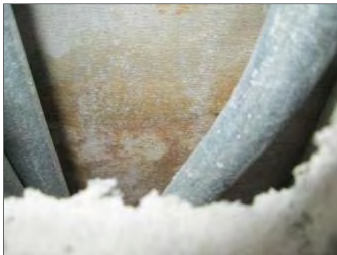
Photo 21 – Range L, water damage and mould growth inside wall cavity.
