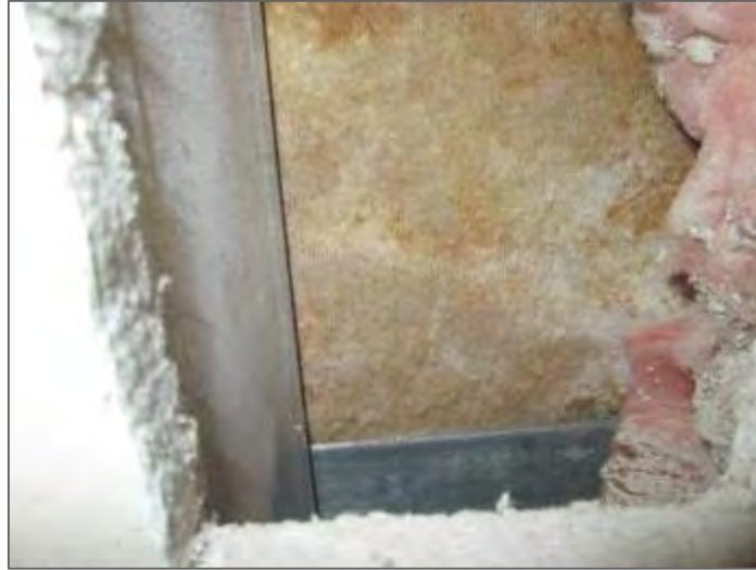
Photo 11 – Range F, damage to drywall inside wall cavity.
