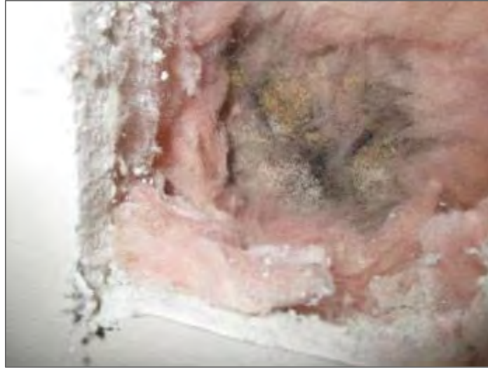
Photo 7 – Range D, mould growth inside wall cavity.
