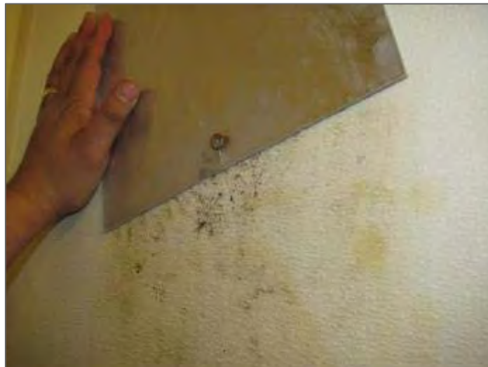
Photo 14 – Range G, mirror mounted in shower, mould growth behind mirror.
