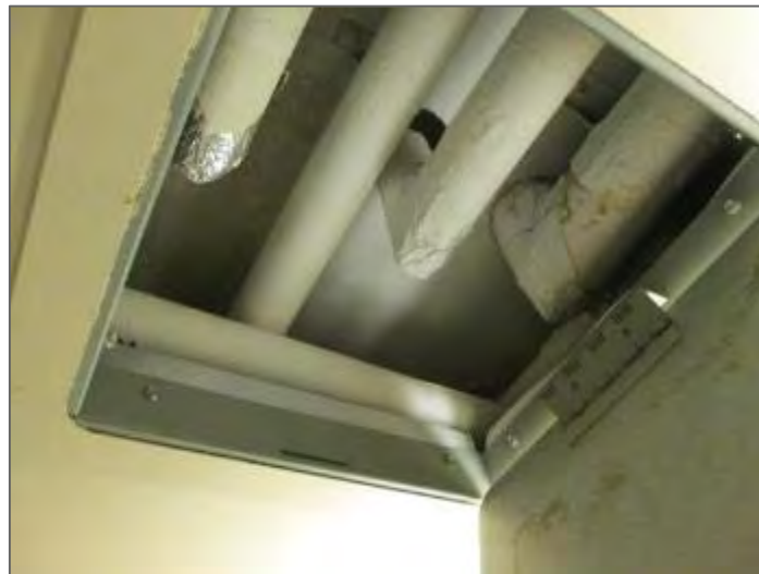
Photo 16 – Range H, typical pipe chase in washroom.
