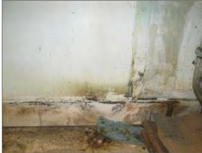
Photo 23 – Range M, mould growth and water damage under kitchen sink.
