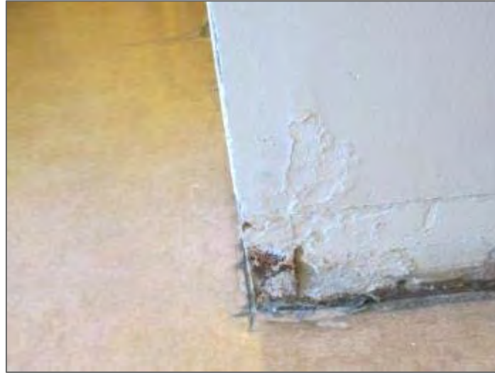
Photo 15 – Range H, rust forming on corner of drywall and paint bubbling from moisture.
