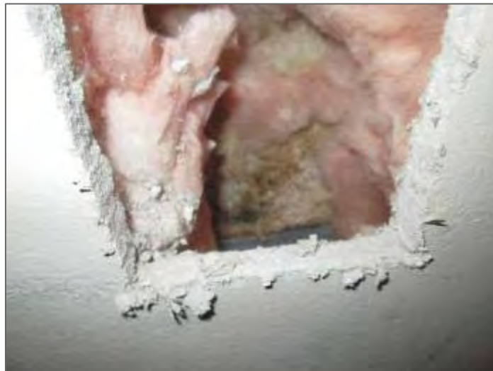
Photo 4 – Range B, mould growth inside wall cavity.
