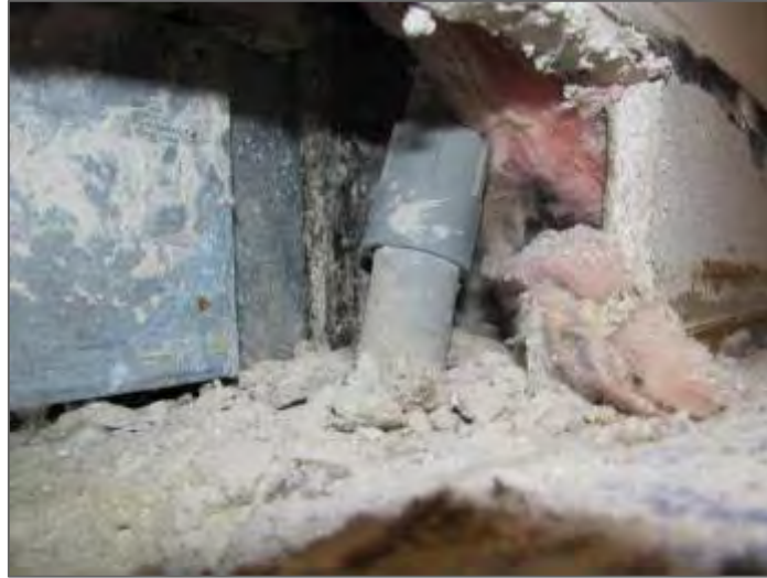
Photo 9 – Range E, mould growth inside wall cavity.
