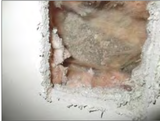
Photo 5 – Range C, typical conditions inside wall cavity surrounding showers.
