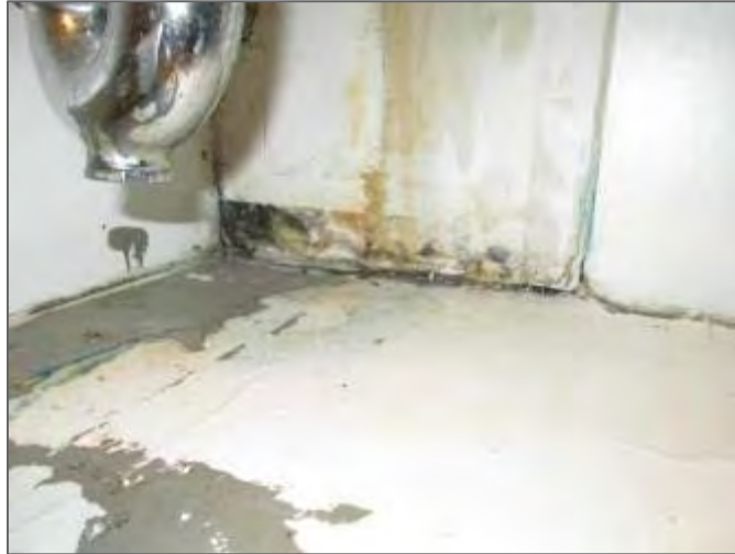
Photo 17 – Range J, mould growth under kitchen sink.
