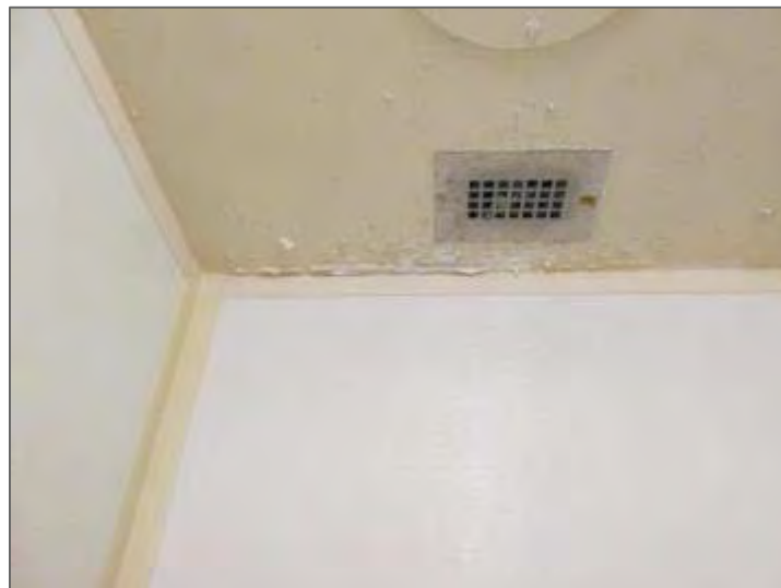
Photo 2 – Range A, typical view of shower ceiling, peeling paint and dusty exhaust vent.
