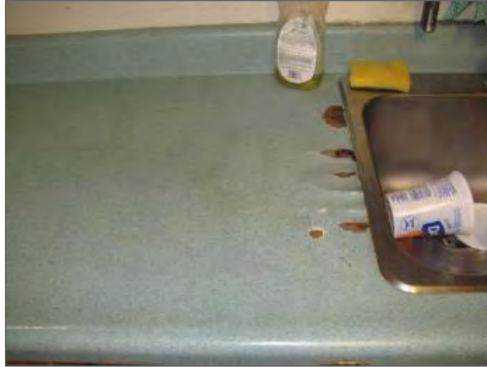
Photo 13 – Range G, water damaged counter top in kitchen.
