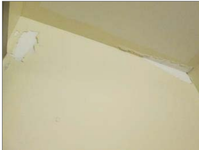
Photo 6 – Range C, paint peeling off of walls in washroom.
