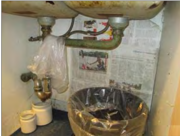
Photo 1 – Range A, conditions under sink, mould growth discovered under newspaper, tray and jars set to collect water dripping from pipes.
