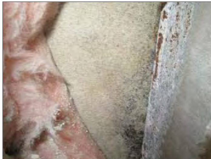
Photo 24 – Range M, mould growth and rusted stud within wall cavity.
