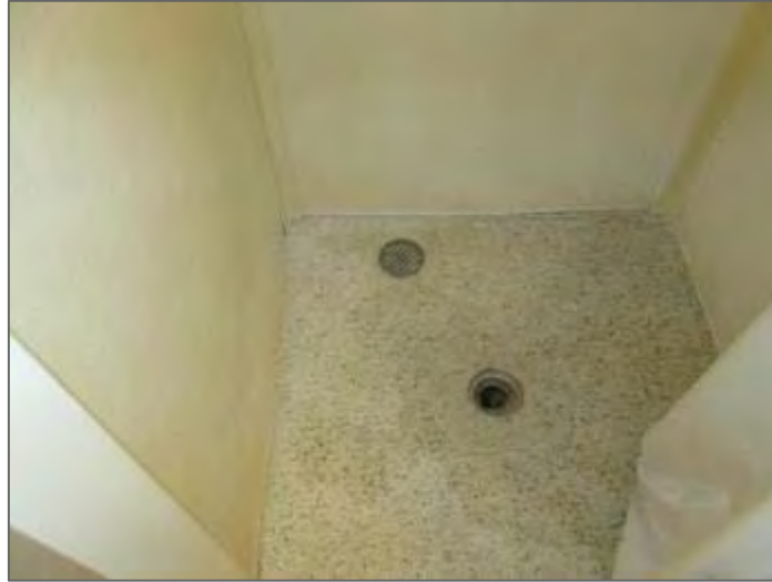
Photo 3 – Range B, bottom of shower, water pooling near drain.
