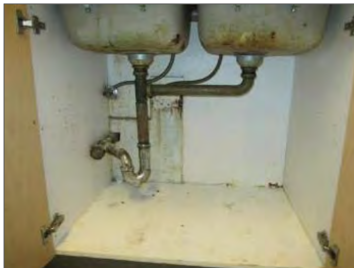
Photo 22 – Range L, water damage and mould growth under kitchen sink.
