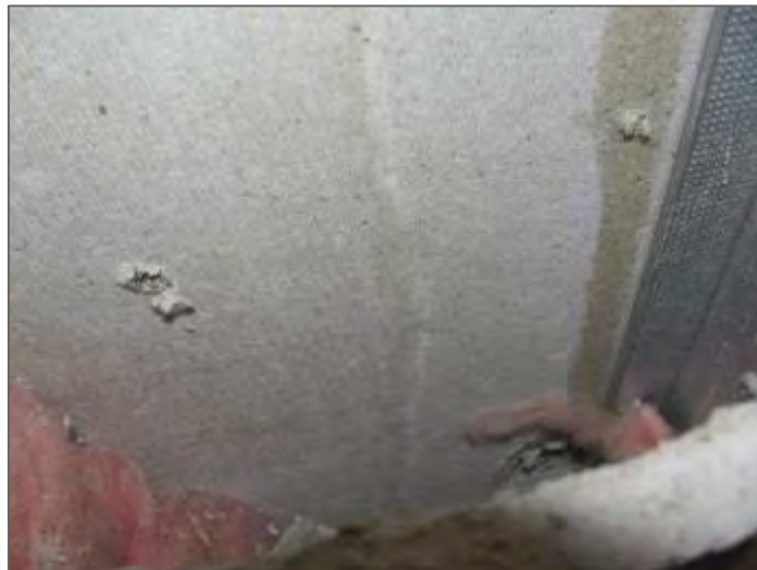
Photo 10 – Range E, visible moisture on drywall inside wall cavity.
