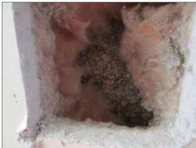
Photo 19 – Range K, mould growth inside wall cavity.
