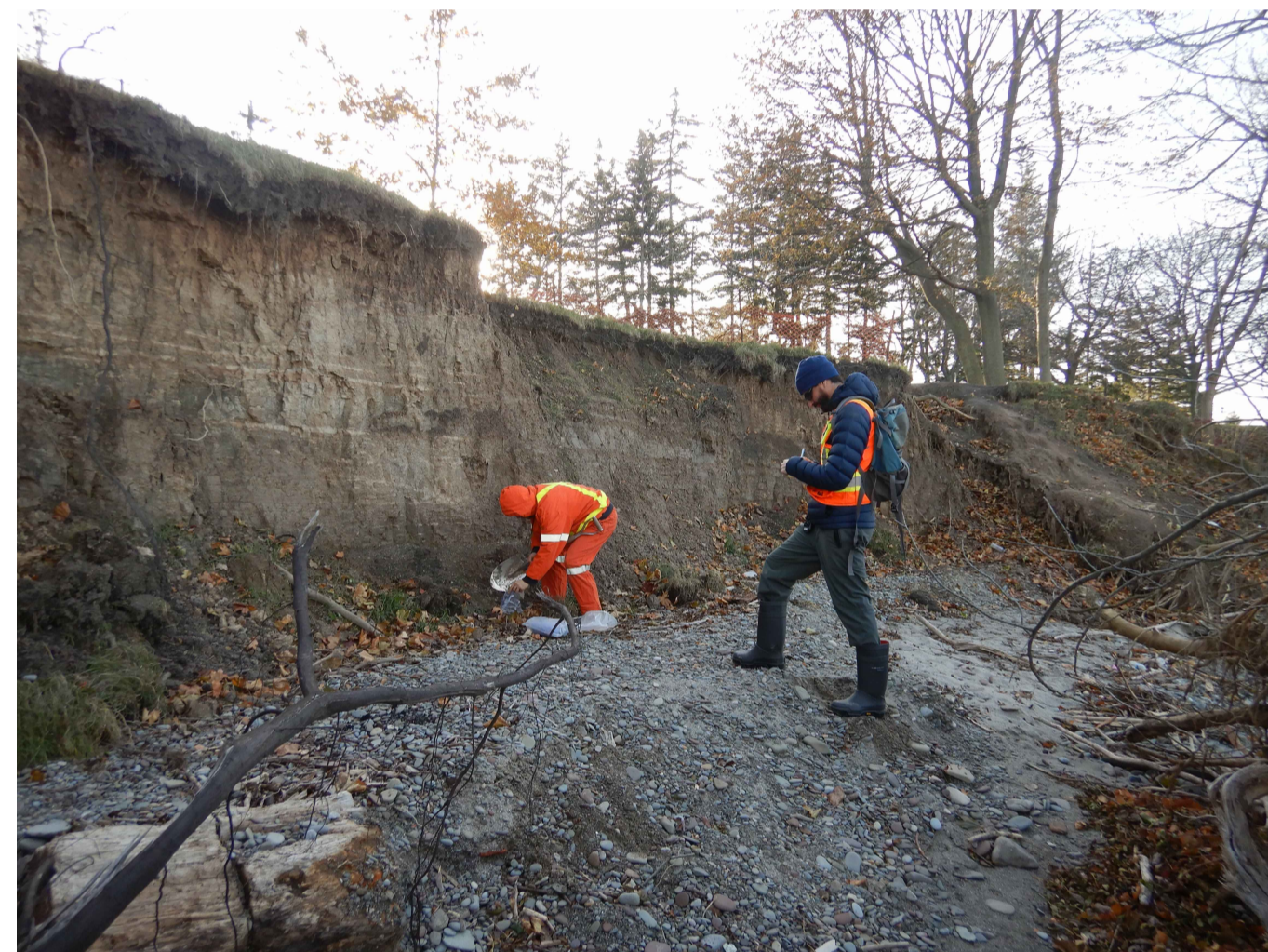
PHOTO 11 - SHORE AND BLUFF NEAR MIDDLE OF SITE, NEAR FROM CHAINAGE 0+040
