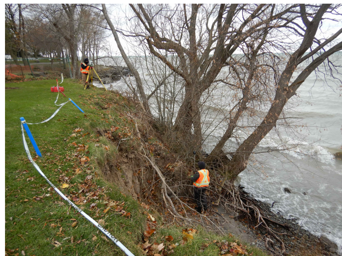
PHOTO 12 - TOP OF BANK NEAR CHAINAGE 0+060
