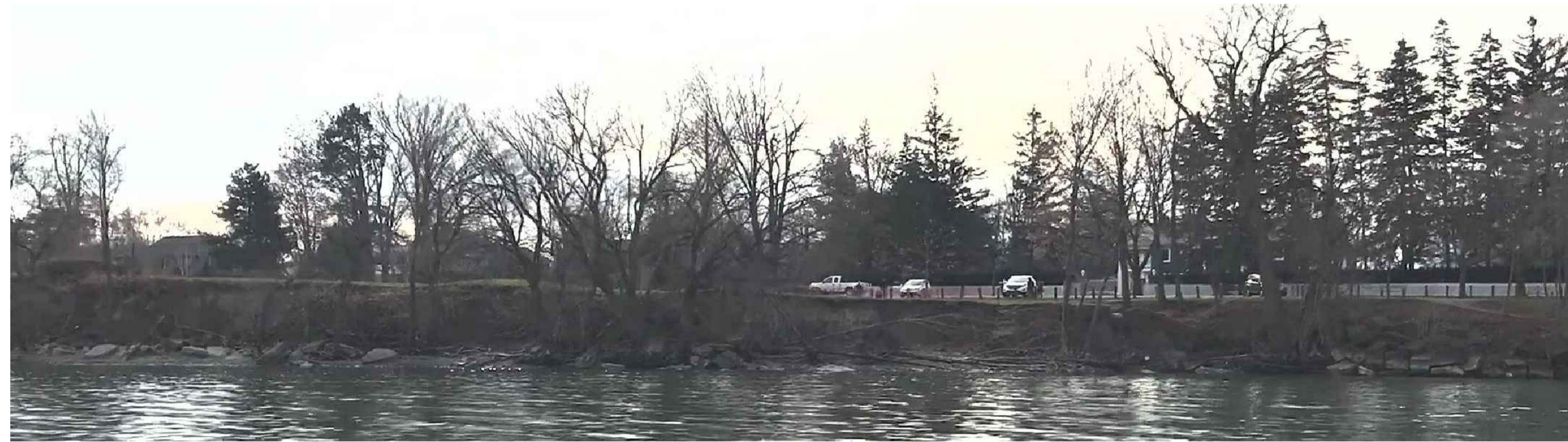
PHOTO 2 - VIEW OF WORK SITE FROM LAKE ONTARIO
