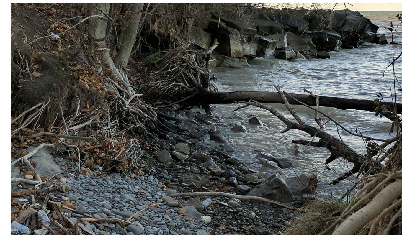
PHOTO 6 - WEST LIMIT OF WORK SITE ADJACENT TO EXISTING SHORE ARMOUR ROCK
