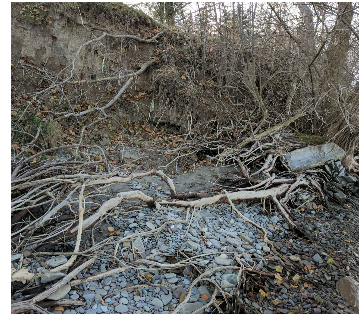
PHOTO 13 - SHORE NEAR CHAINAGE 0+070
