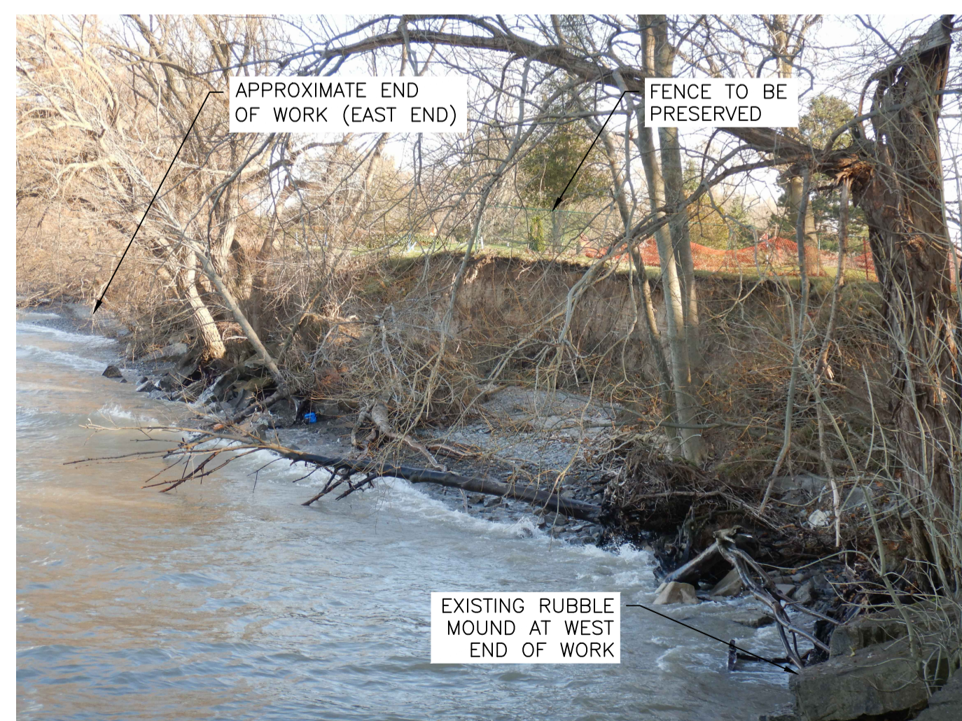
PHOTO 9 - OVERALL VIEW OF SHORELINE IN WORK SITE
