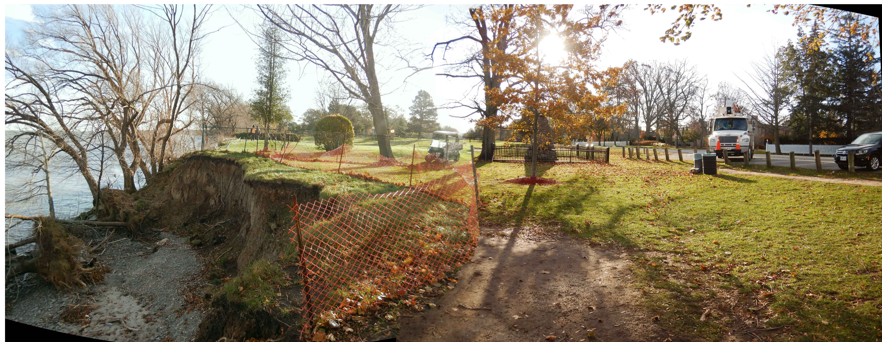
PHOTO 3 - VIEW OF WORK SITE NEAR NORTH END OF PARKING LOT
