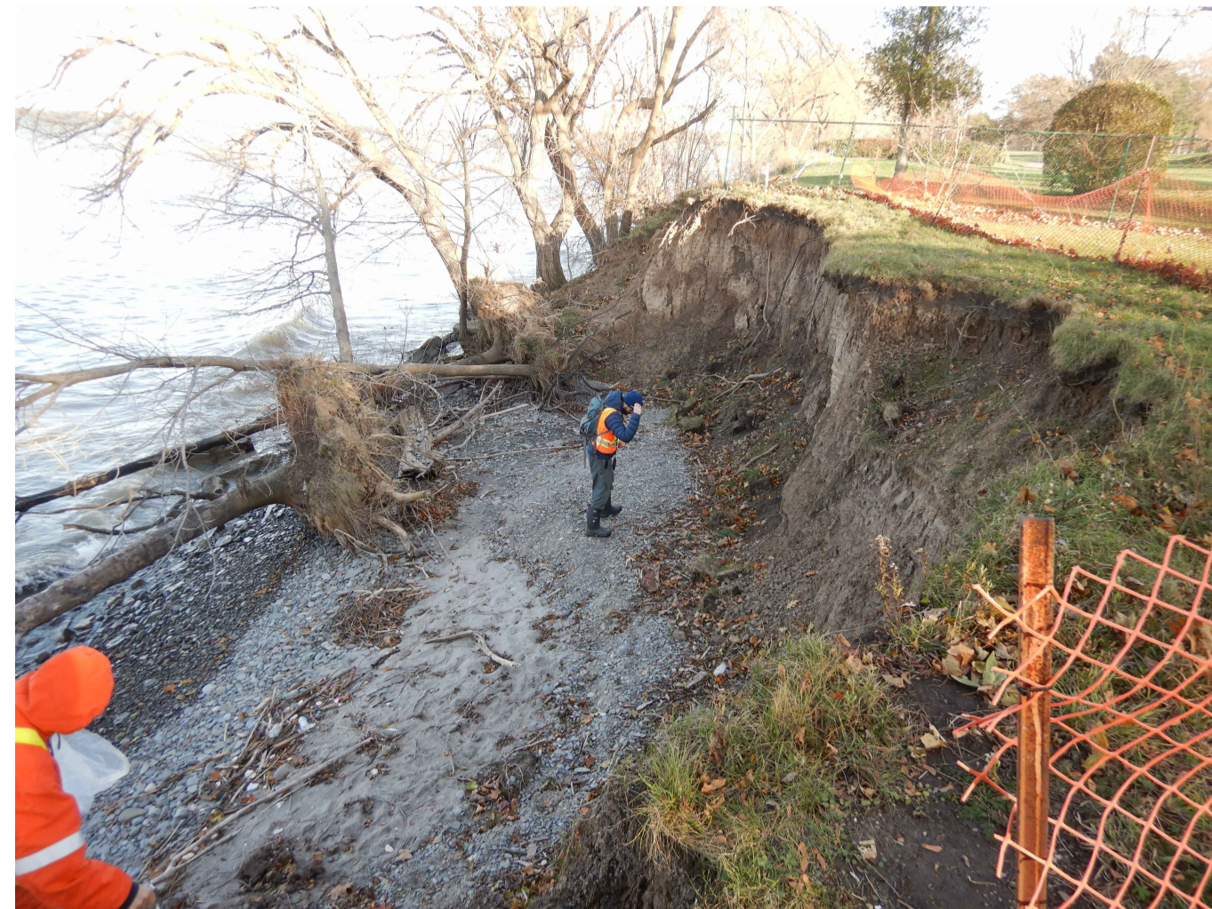
PHOTO 10 - SHORE AND BLUFF NEAR MIDDLE OF SITE, FROM CHAINAGE 0+030
