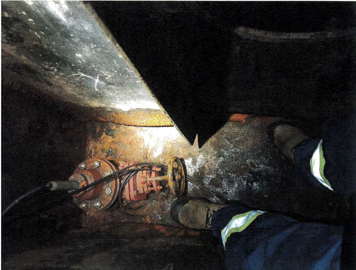
Photograph 8 – View of transverse floor plate in transducer compartment. Buckling of lower edge of floor plate consistent at each frame in way of damage.
